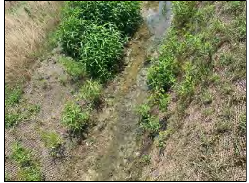
Area of Removed Culvert
