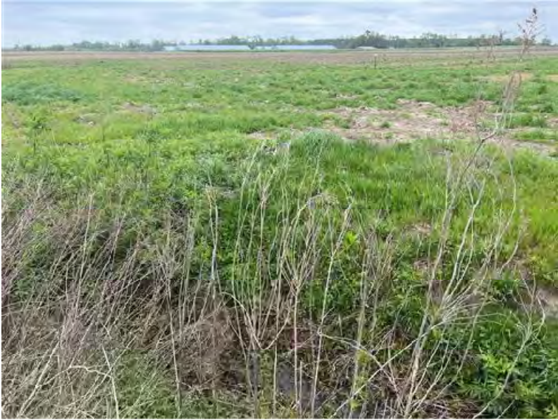
First Hydrant Removed on J1
