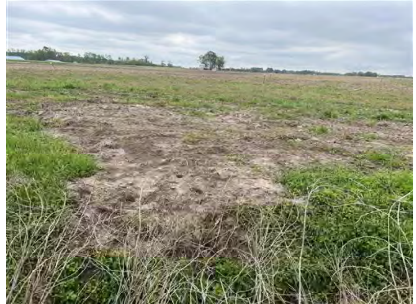
Second Hydrant Removed on J1
