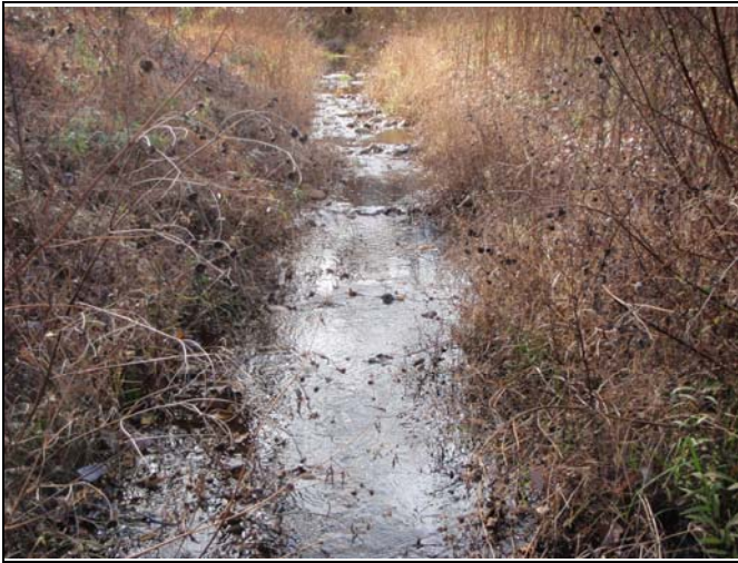
Photo Point 118 – Constructed Riffle, UT5 Reach 1
