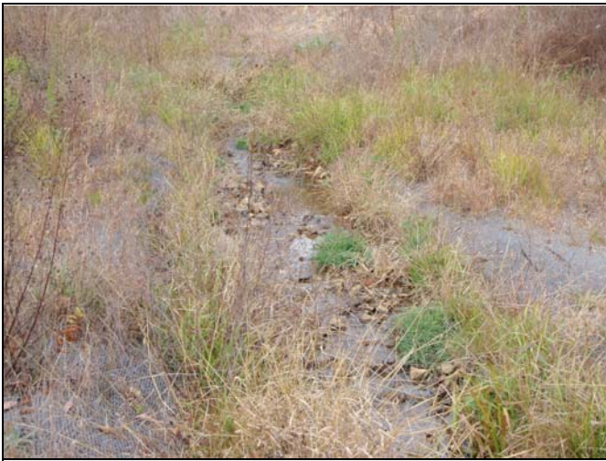
Photo Point 74 – Constructed Riffle, UT1 Reach 1
