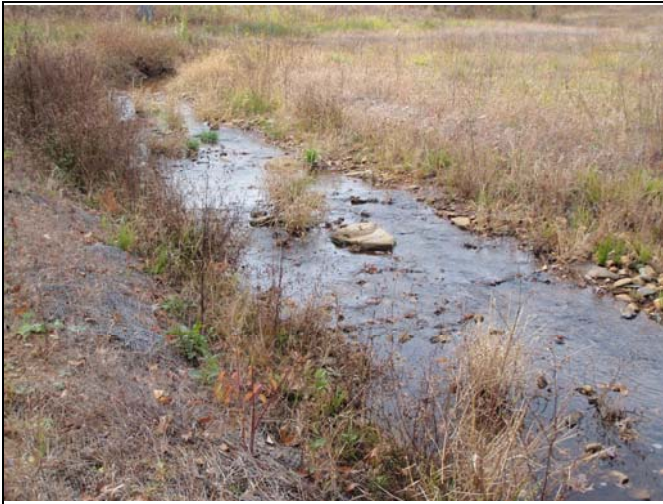
Photo Point 27 – Constructed Riffle, UT1 Reach 4
