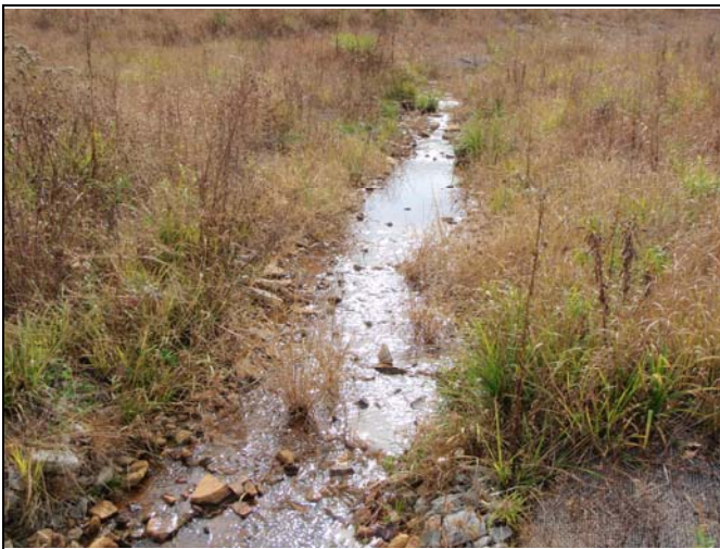
Photo Point 59 – Constructed Riffle, UT1 Reach 2
