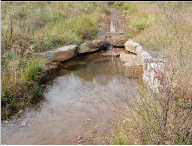
Photo Point 32 – Cross Vane, UT1 Reach 3
