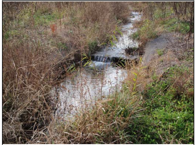
Photo Point 109 – Constructed Riffle, UT5 Reach 1 End
