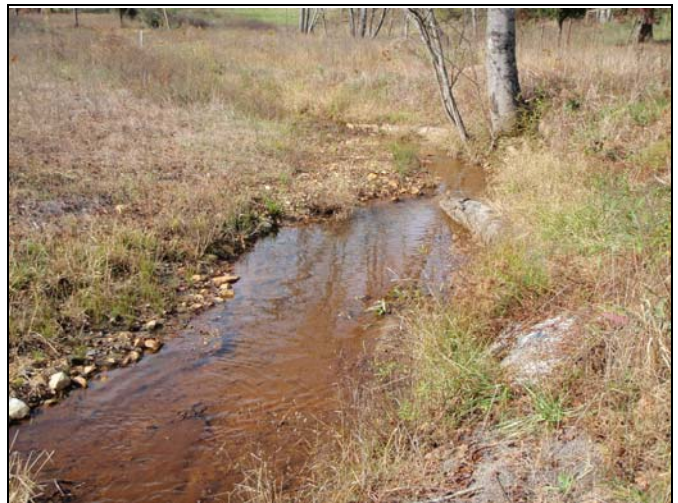
Photo Point 7 and 8 – Constructed Riffle, UT1 Reach 4
