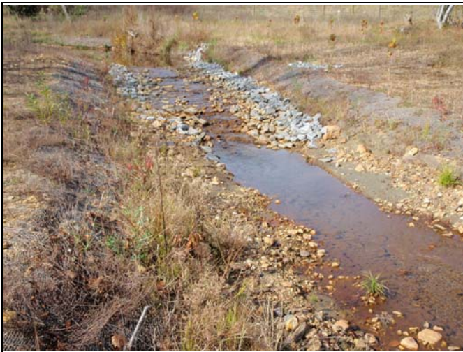
Photo Point 11 – Constructed Riffle, UT1 Reach 4
