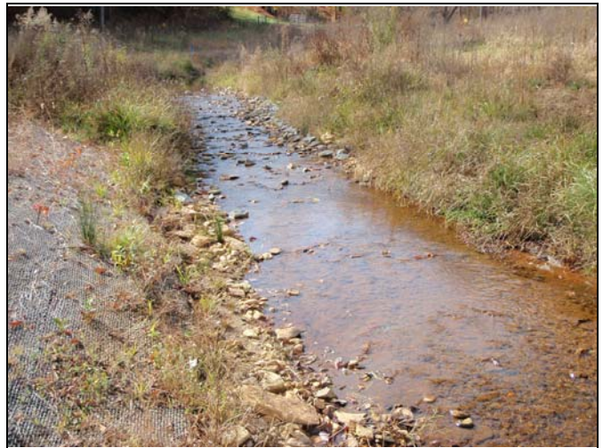
Photo Point 12 – Constructed Riffle, UT1 Reach 4
