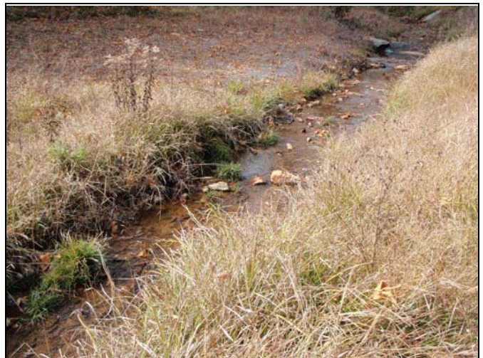
Photo Point 48 – Constructed Riffle, UT1 Reach 3
