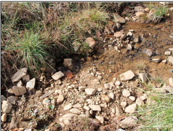
Photo Point 35 – Step Pool Piping, UT1 Reach 3
