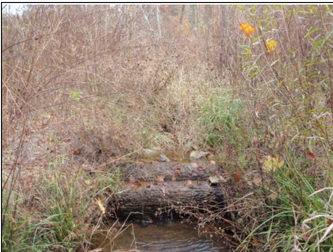
Photo Point 133 – Log Step Pool, UT6
