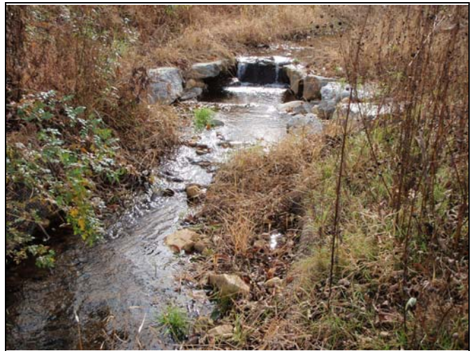
Photo Point 111 – Cross Vane, UT5 Reach 1
