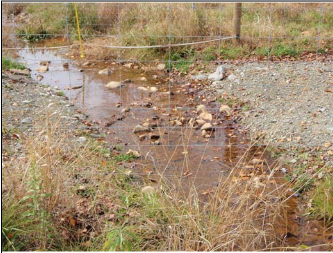
Upstream of Photo Point 66 – Constructed Riffle/Stream Crossing, UT1 Reach 2
