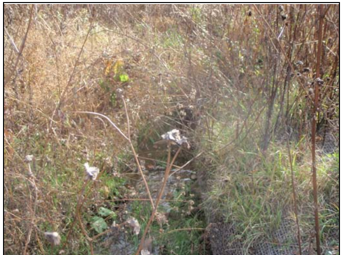
Photo Point 121 – Constructed Riffle, UT6
