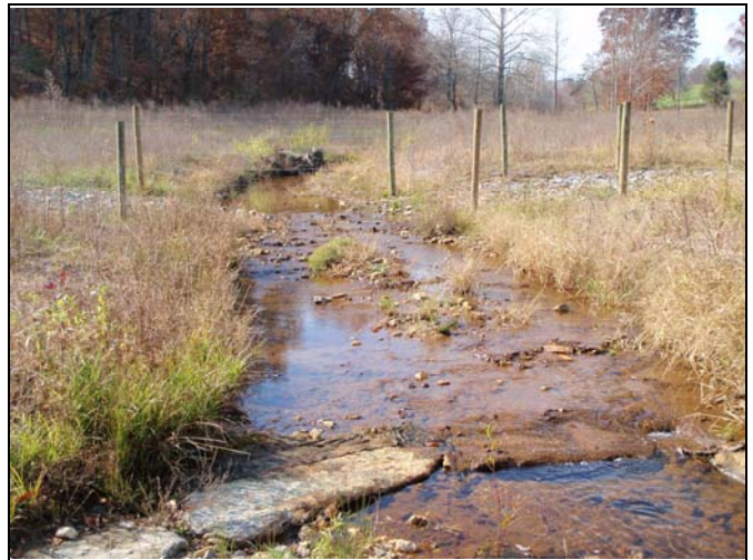
Photo Point 5 – Constructed Riffle, UT1 Reach 4
