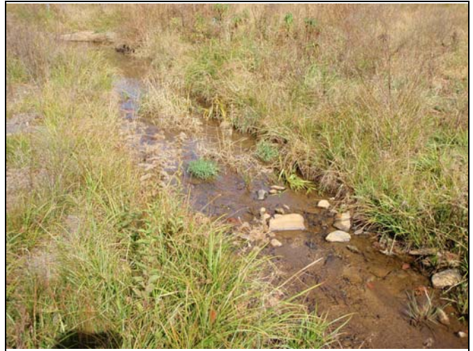
Photo Point 38 – Constructed Riffle, UT1 Reach 3
