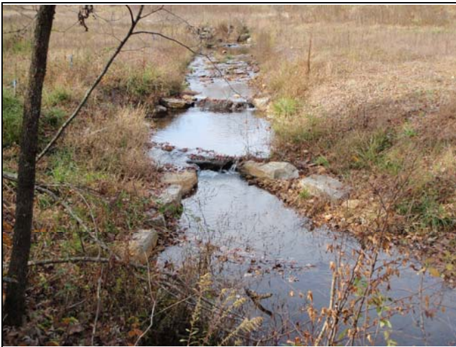
Photo Point 23 – Rock J-Hook, UT1 Reach 4
