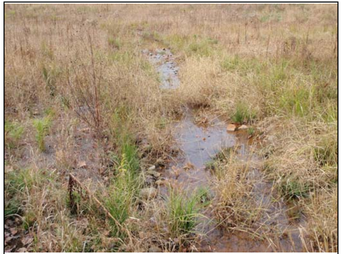
Photo Point 58 – Constructed Riffle, UT1 Reach 2
