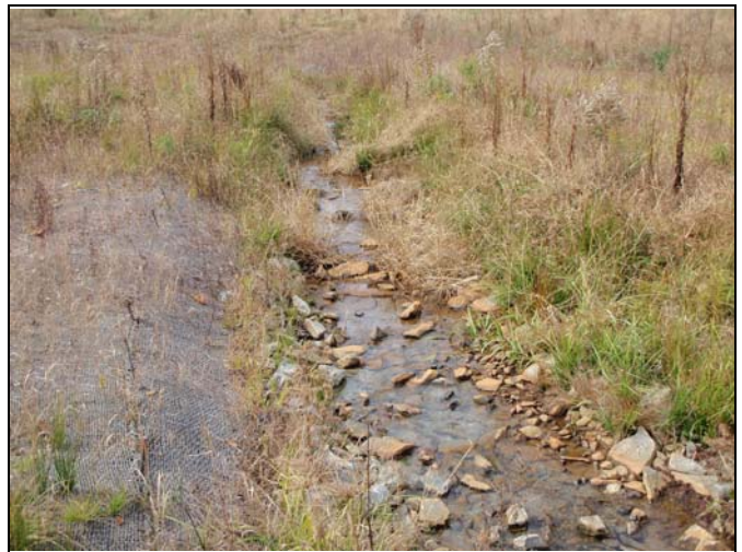
Photo Point 60 – Constructed Riffle, UT1 Reach 2
