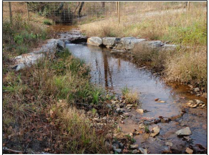
Photo Point 16 – Cross Vane, UT1 Reach 4
