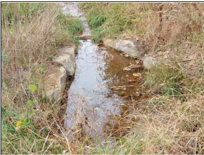
Photo Point 81 – Cross Vane, UT1 Reach 1
