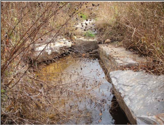
Photo Point 104 – Rock J-Hook, UT5 Reach 2
