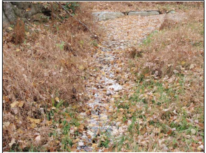
Photo Point 91 – Constructed Riffle, UT1 Reach 1
