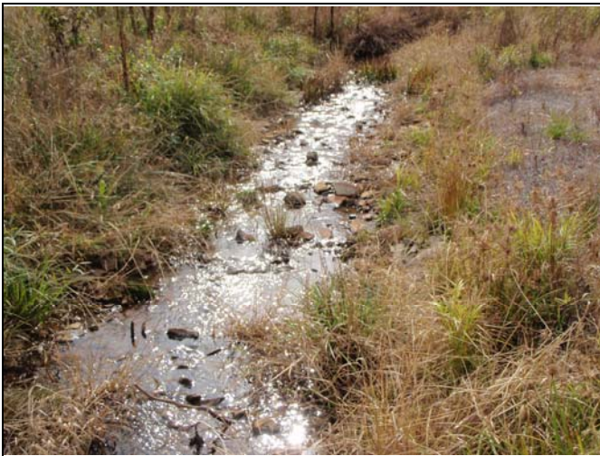
Photo Point 63 – Constructed Riffle, UT1 Reach 2
