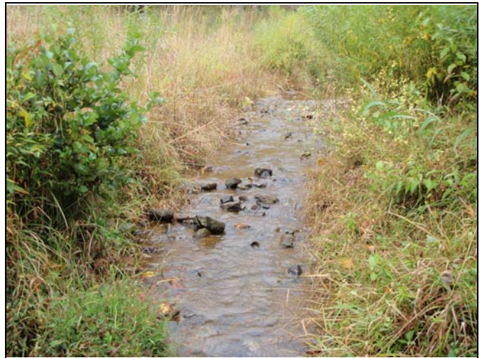
Photo Point 9 – Constructed Riffle, UT1 Reach 4
