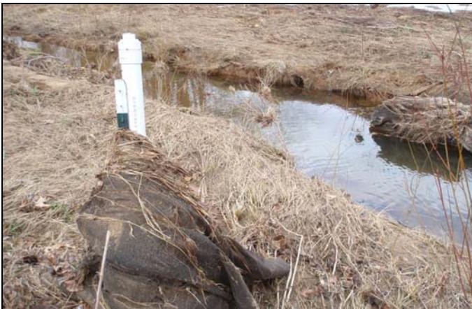
Looking at debris line on crest gauge at UT5_R2 after January 2010 storm event
