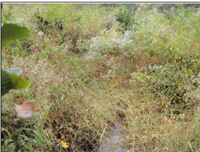
Photo Point 70 – Constructed Riffle, UT1 Reach 2 Begin
