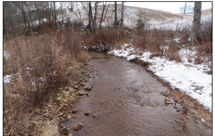
AFTER: Re-shaped riffle along UT1_R4 near station 59+50
