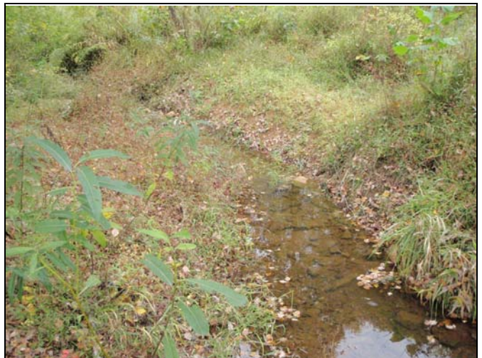
Photo Point 118 – Constructed Riffle, UT5 Reach 1
