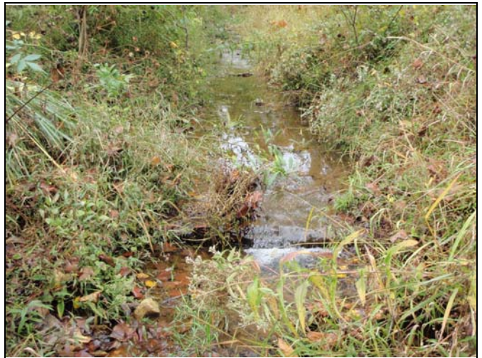
Photo Point 116 – Constructed Riffle, UT5 Reach 1
