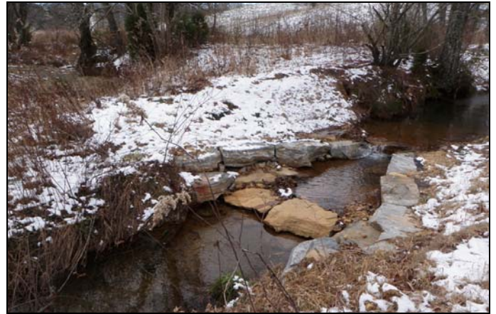
AFTER: Installed cross vane to increase bed/bank stability and improve habitat
