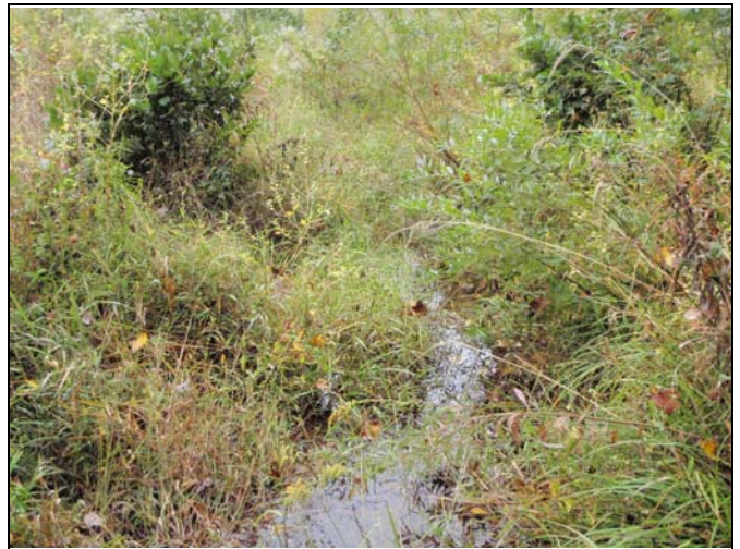
Photo Point 69 – Constructed Riffle, UT1 Reach 2
