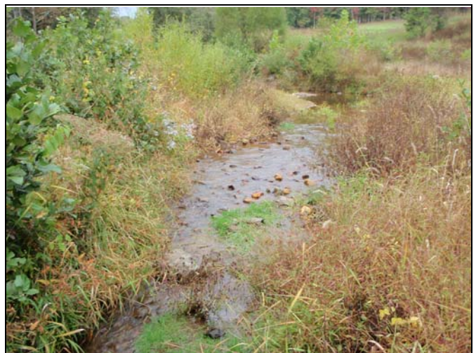
Photo Point 11 – Constructed Riffle, UT1 Reach 4
