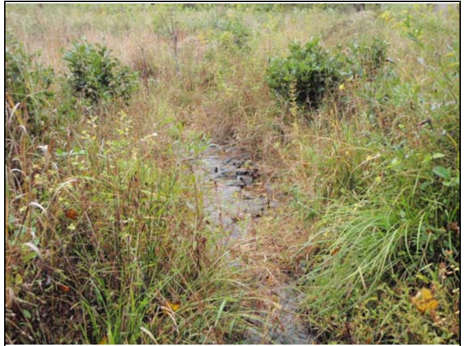
Photo Point 55 – Constructed Riffle, UT1 Reach 2
