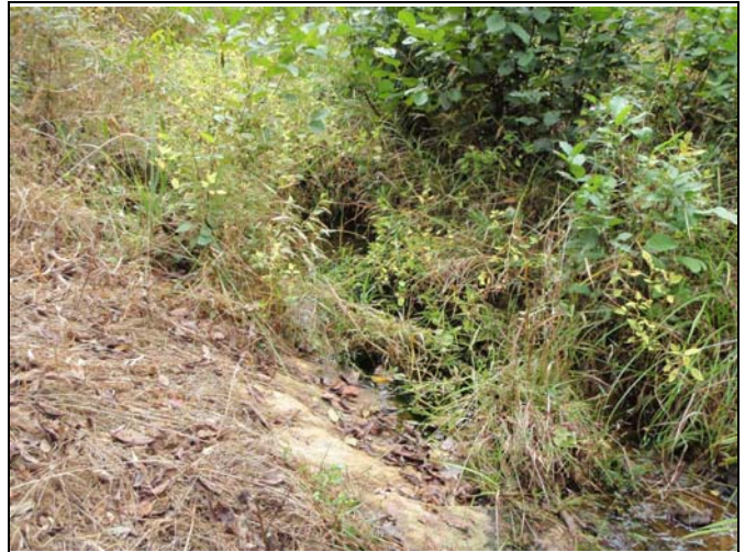
Photo Point 140 – Constructed Riffle, UT6
