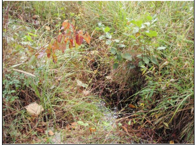
Photo Point 132 – Constructed Riffle, UT6
