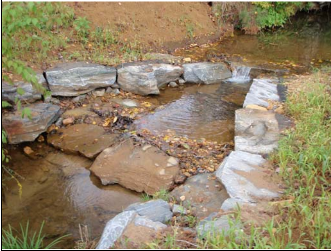
Photo Point 30 – Cross Vane, UT1 Reach 4 End
