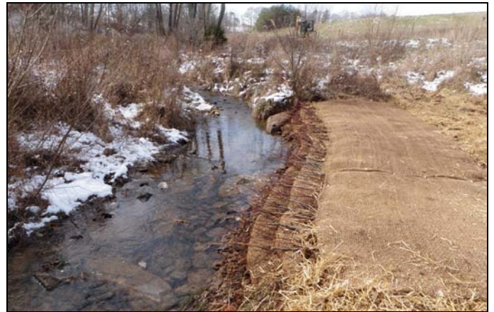
AFTER: Installed geolift, view is upstream immediately after bank repair
