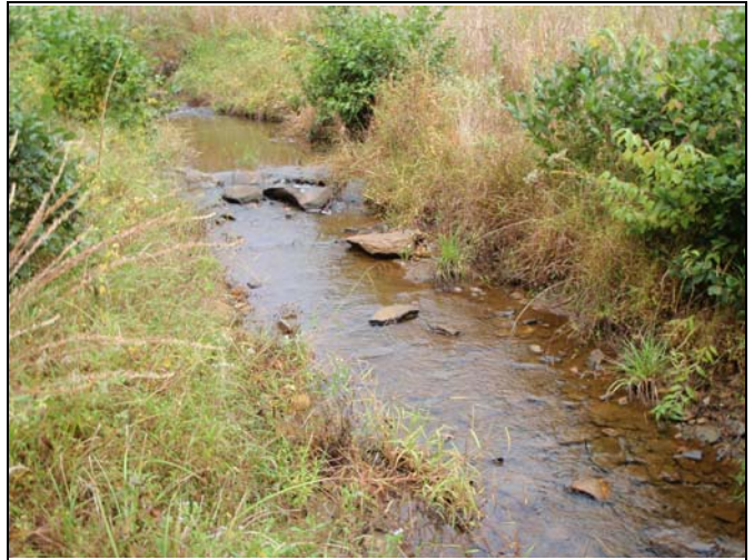
Photo Point 25 – Constructed Riffle, UT1 Reach 4
