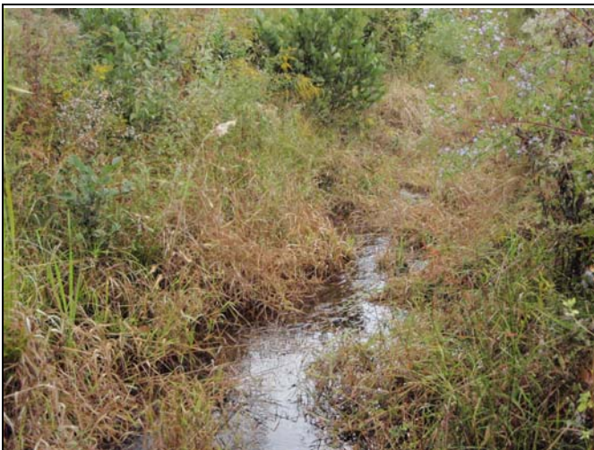
Photo Point 46 – Constructed Riffle, UT1 Reach 3
