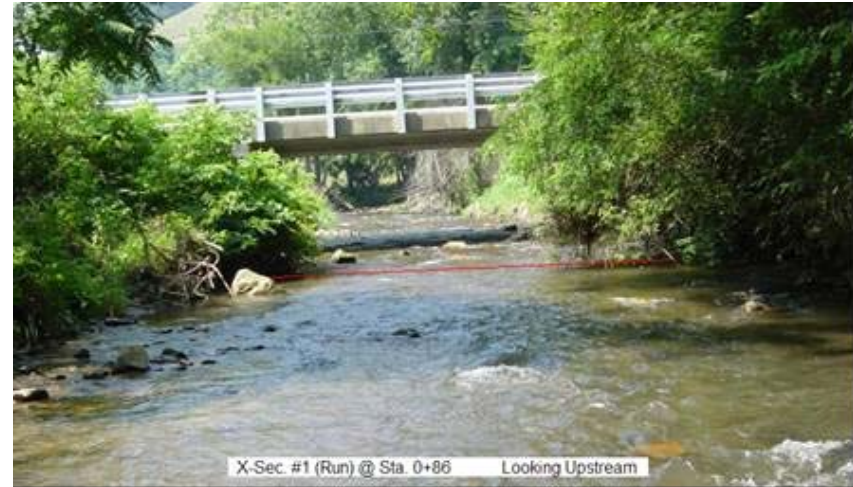
A1.2.—Cross-section 1, sta. 0+86, run, looking upstream.
