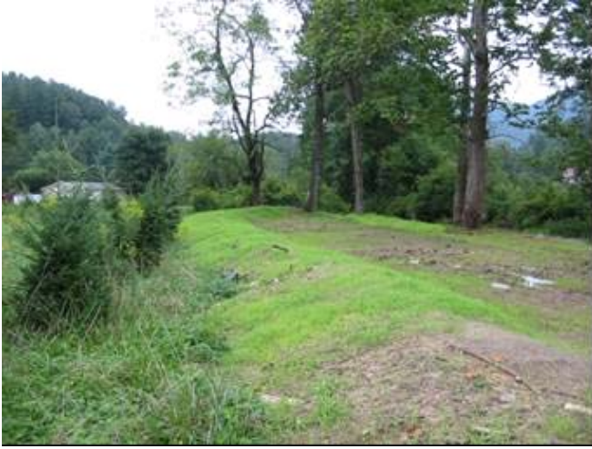
Photo station 4, left bank facing downstream, 5 Sep 2006.
