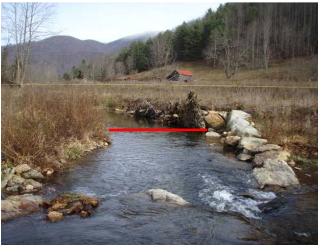
Cross-section 4, facing downstream, 5 Dec 07.
