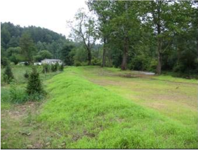
Photo station 3, left bank facing downstream, 5 Sep 2006.
