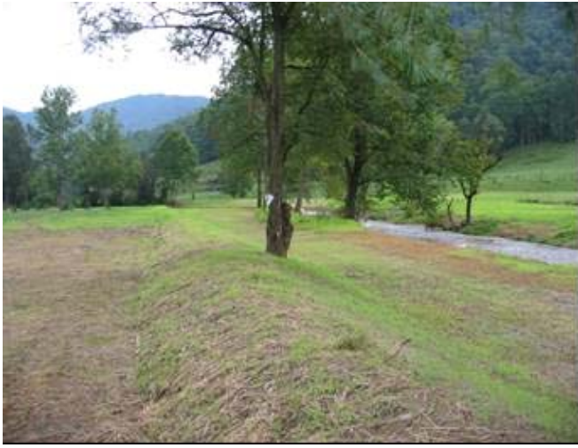
Photo station 1, left bank facing downstream, 5 Sep 2006.
