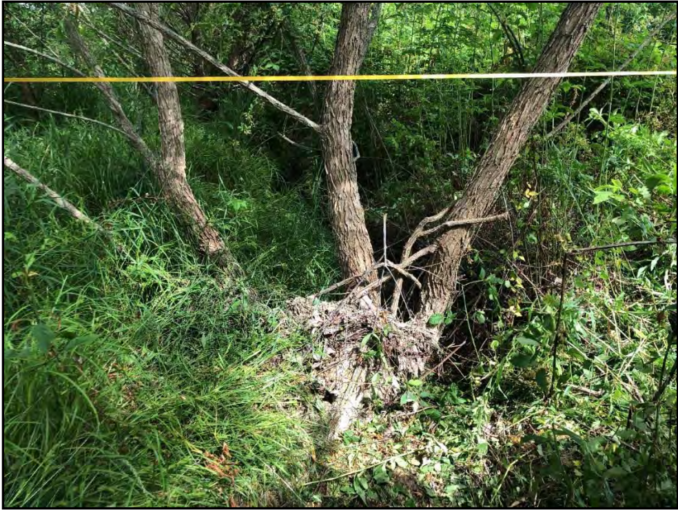
Project Reach UT2-A – Permanent Photo Station 17 Station 2+62 – Looking Downstream – 6/3/2021
