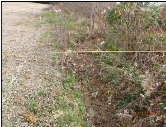
Facing downstream on UT1-R2 (P1 Restoration). 12/11/12
