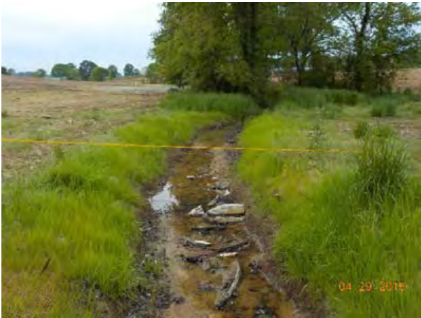
UT1-A STA 2+00 Looking Downstream (4/29/2015)
