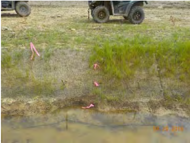
Bank Pin Array 3 UT1-2 STA 18+75 (4/29/2015)
