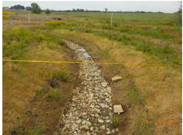
UT1-B STA 9+86 Looking Downstream (4/29/2015)
