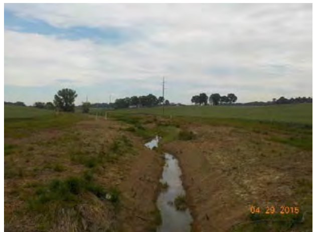
UT1-4 STA 47+20 Looking Upstream (4/29/2015)
