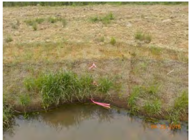
Bank Pin Array 6 UT1-4 STA 40+10 (4/29/2015)
