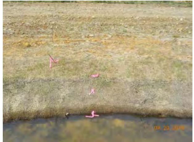
Bank Pin Array 4 UT1-3 STA 28+75 (4/29/2015)
