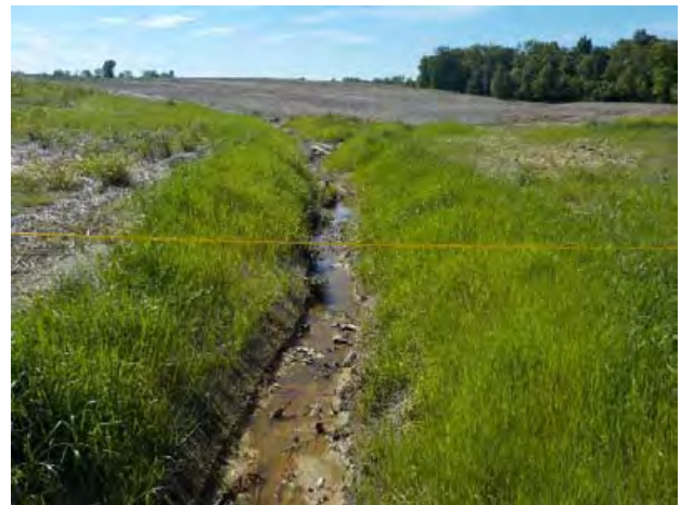
UT2-A STA 1+22 Looking Upstream (4/29/2015)
