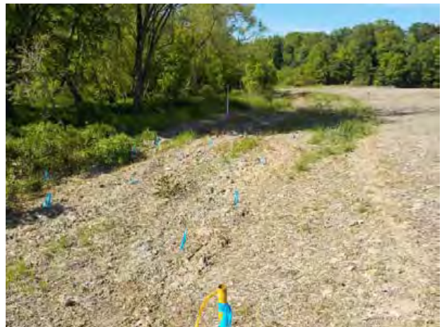
UT2-1 STA 4+50 Looking Upstream (4/29/2015)
