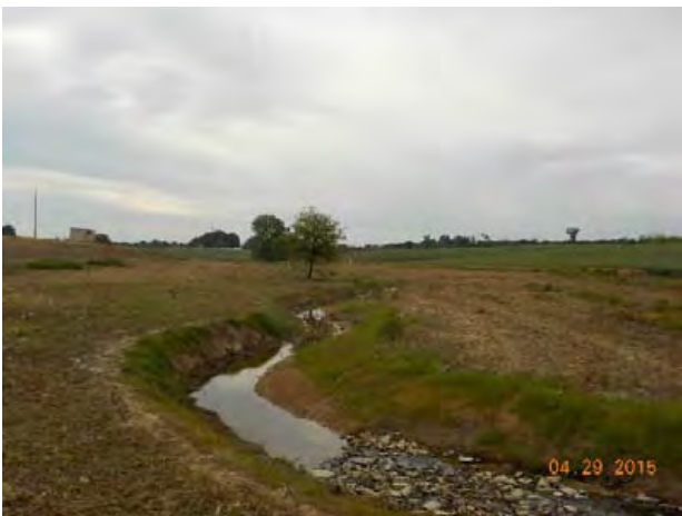
UT1-3 STA 27+50 Looking Downstream (4/29/2015)
