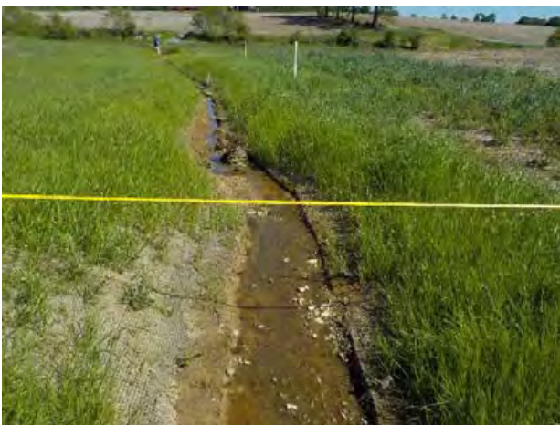
UT2-A STA 2+62 Looking Downstream (4/29/2015)
