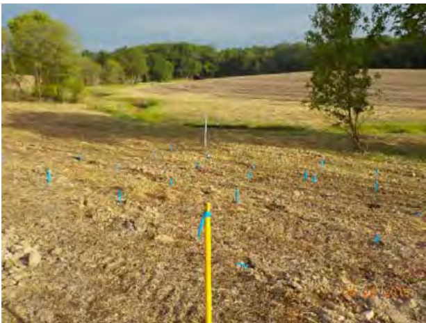
UT1-2 STA 21+50 Looking Upstream (4/29/2015)
