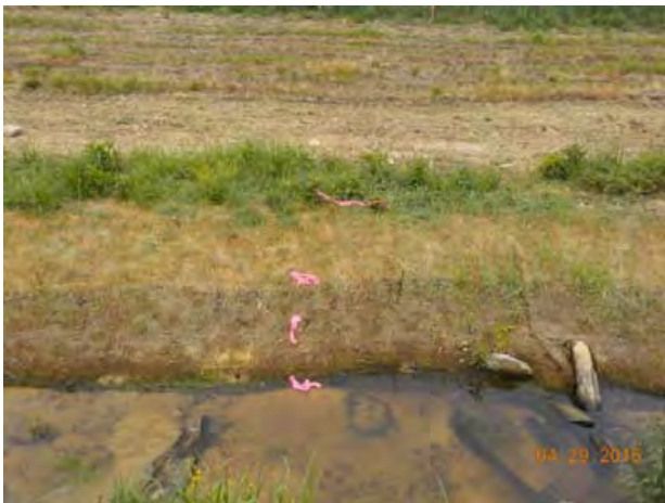
Bank Pin Array 5 UT1-C STA 4+60 (4/29/2015)
