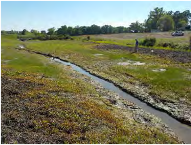
UT2-2 STA 7+59 Looking Downstream (4/29/2015)
