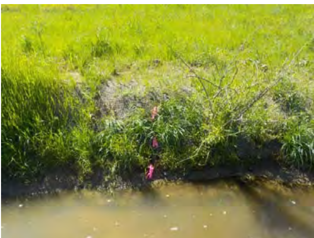
Bank Pin Array 1 UT2-2 STA 13+10 (4/29/2015)
