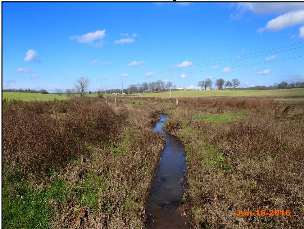
Project Reach UT1-4 – Permanent Photo Station 6 Station 47+20 – Looking Upstream
