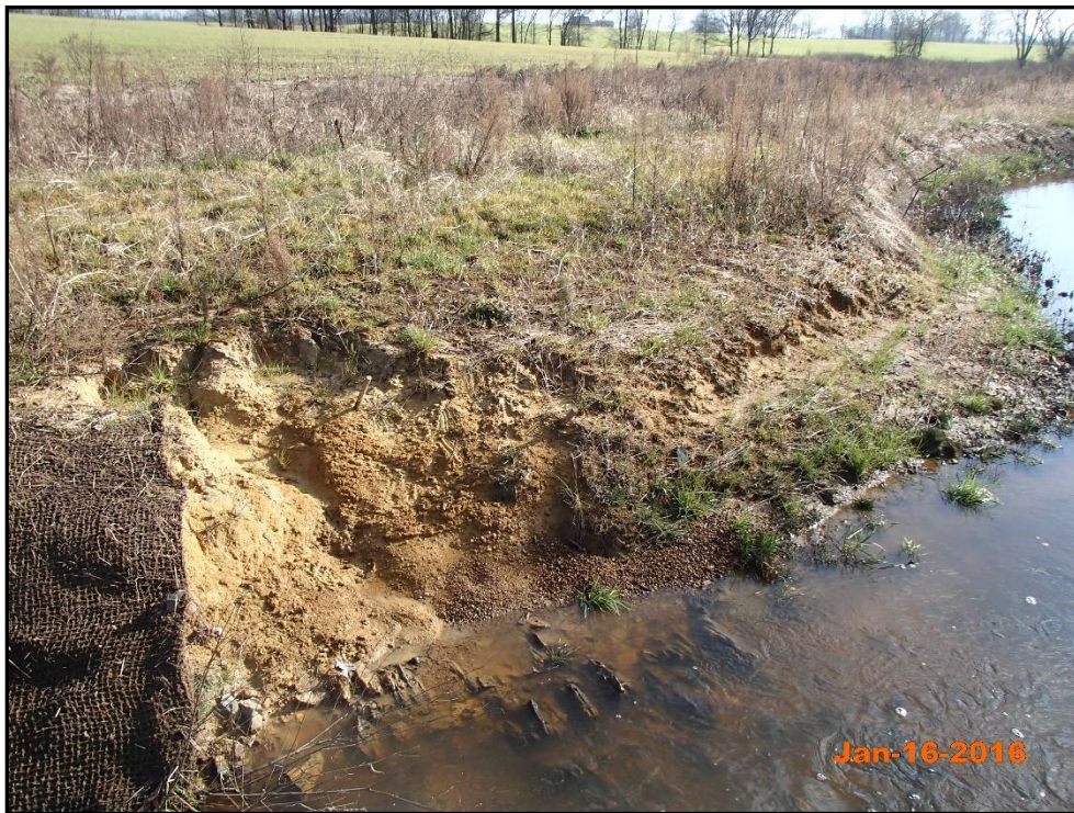
Project Reach UT1-2 – Bank Erosion 18+25 Left Descending Bank
