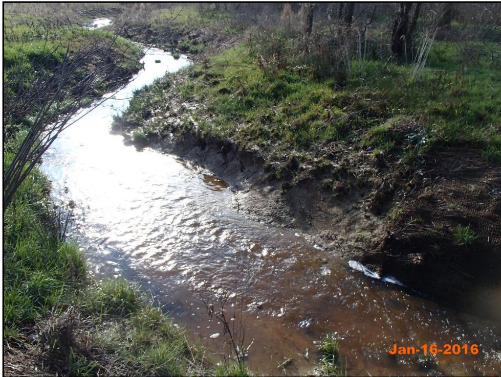
Project Reach UT1-2 – Bank Erosion 15+75 Right Descending Bank
