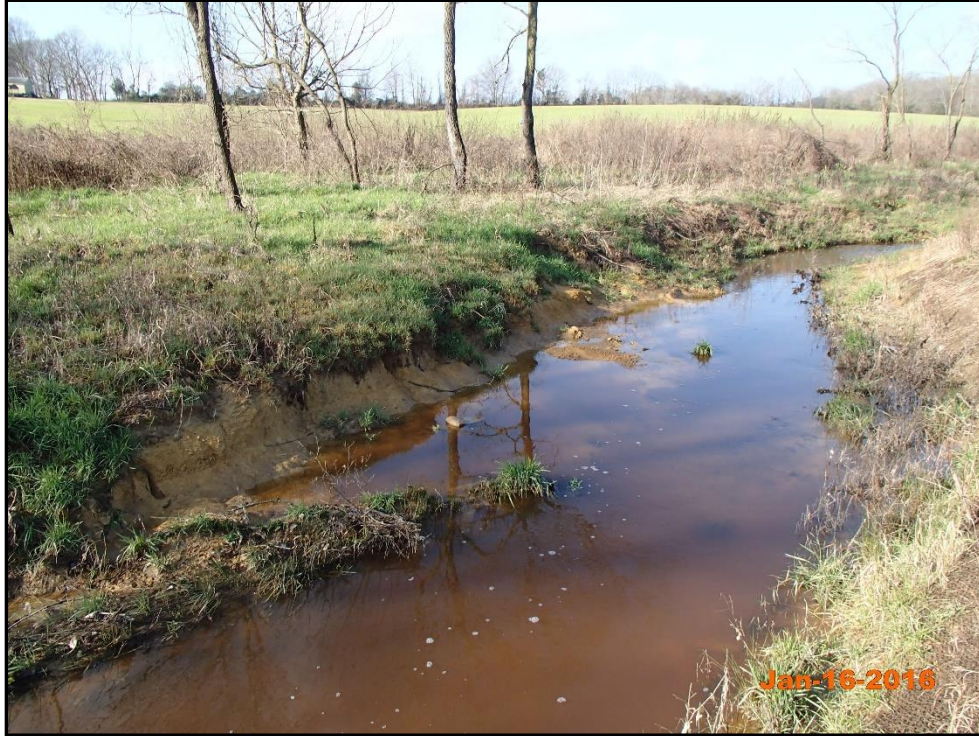
Project Reach UT1-2 – Bank Erosion 19+00 Right Descending Bank
