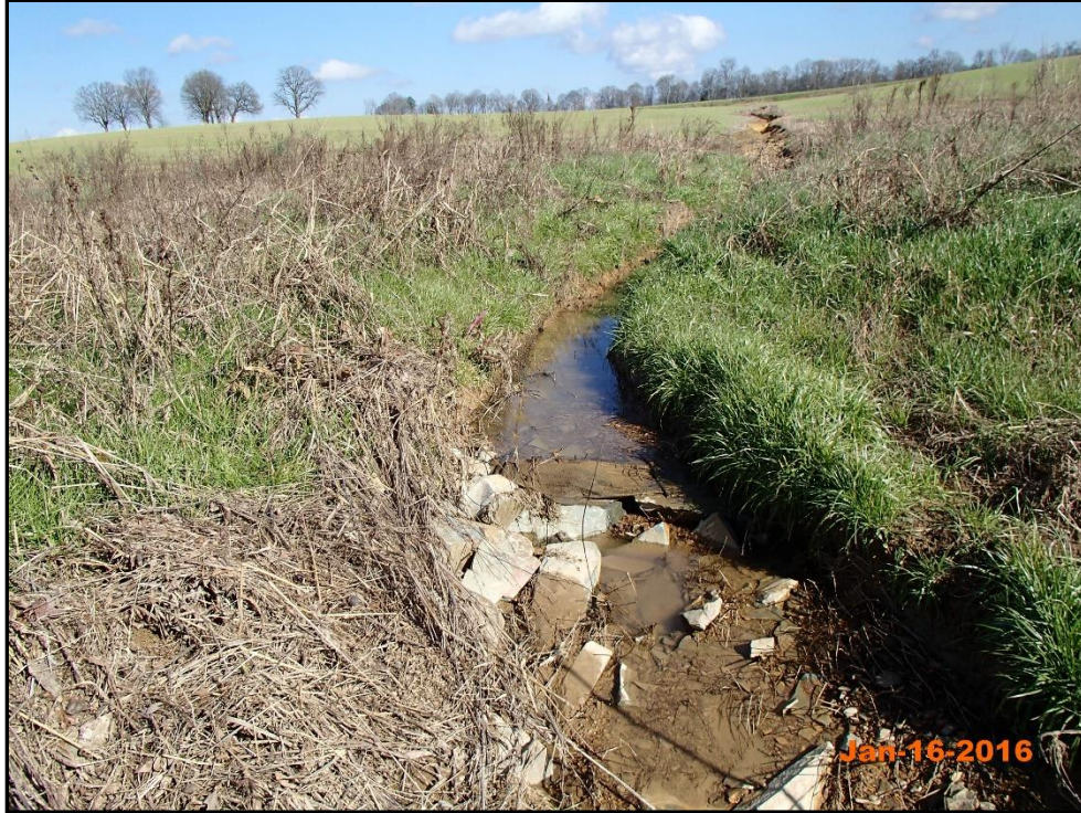
Project Reach UT1-4 – Stressed BMP Structure Left Descending Bank 42+25
