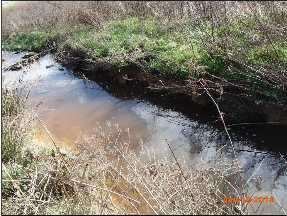
Project Reach UT1-C – Bank Scour 4+00 Right Descending Bank
