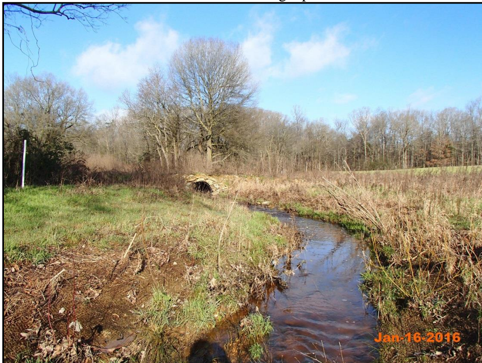
Project Reach UT1-2 – Permanent Photo Station 2 Station 14+58 – Looking Upstream at Crossing
