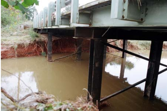
Under the Paint Shop Road Bridge, West.
