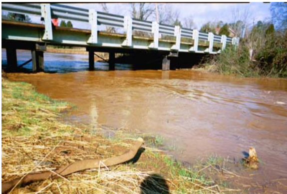
The bridge at Paint Shop Road.
