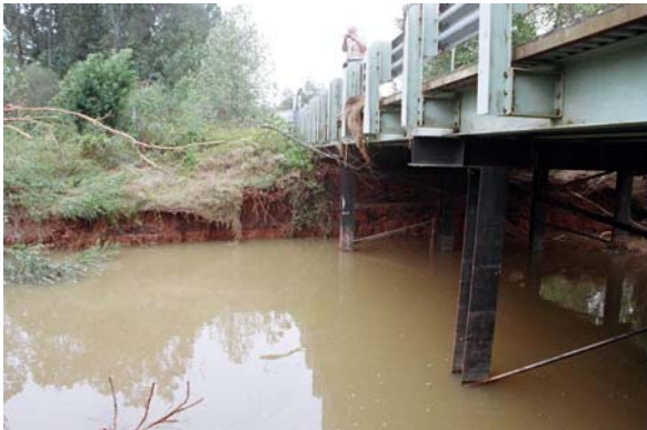
Under the bridge, East.
