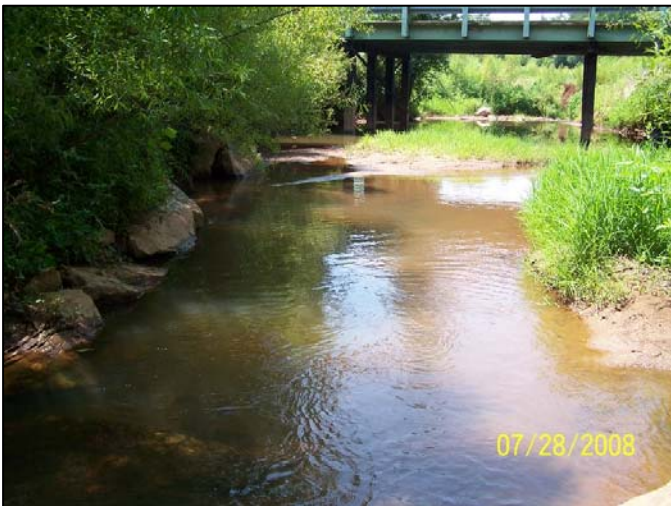
PCCV4U – looking downstream
