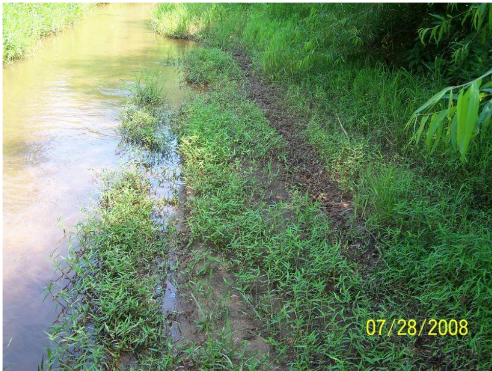
Evidence of 4-Wheeler trespassing, damage to project is minor.
