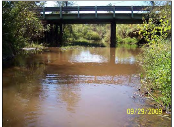
PCCV4U facing downstream
