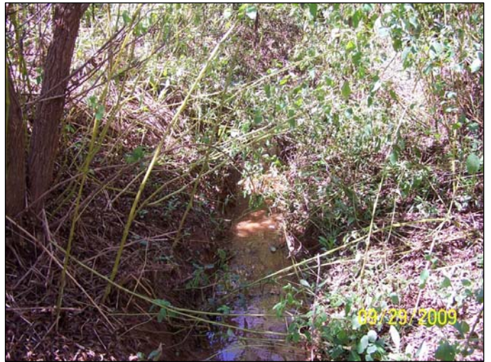
CS UT3 facing downstream
