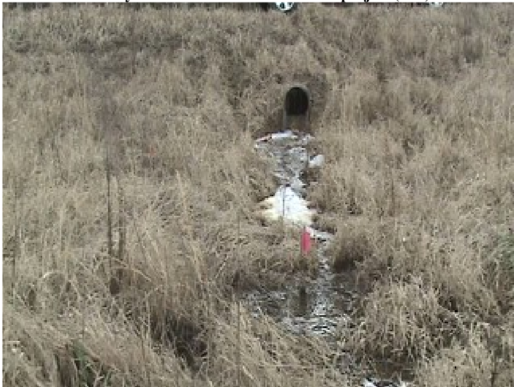
Steady inflow from watershed above project (Dec)
