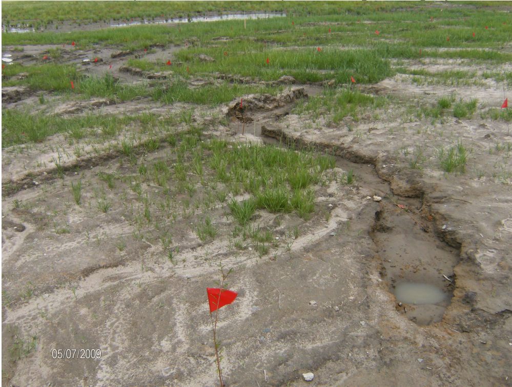
Further early channelization (May) near midpoint of project
