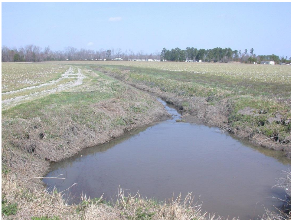
The midpoint of the project became the confluence of the 3 headwaters. View is looking downstream. This area was highly eroded and degraded and prone to sedimentation prior to construction.
