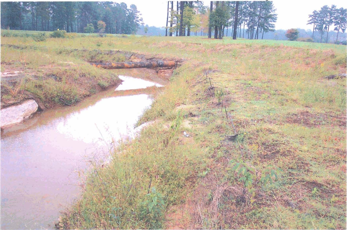
Channel Condition Upstream of Sewer Pipe Appears Stable
