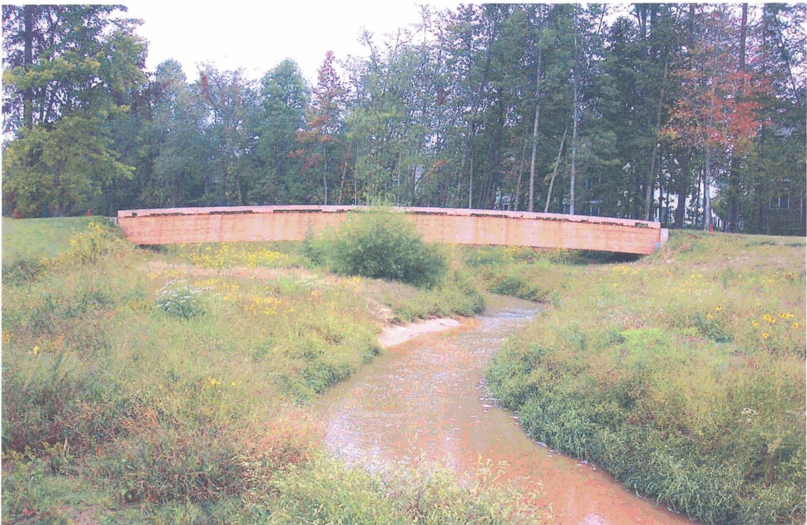
Photograph Taken Below 80-foot Span Bridge
