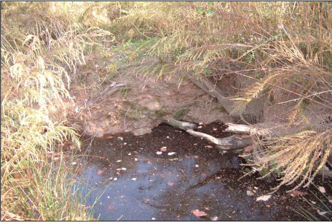
SP7 – Back scour around rootwad and bank erosion. Rootwad partially obscured by coir matting. Photo taken near station 02+10. 11/5/06 - MY 02
