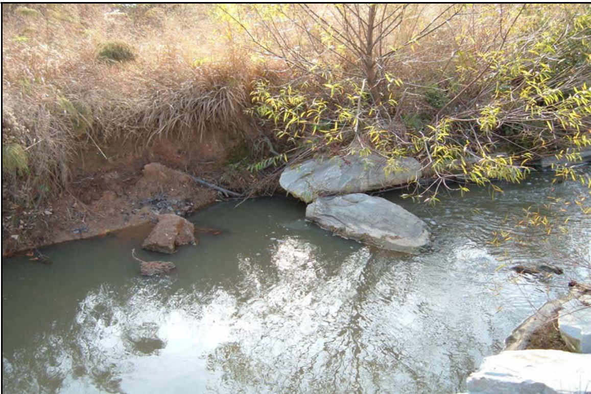
SP4 – Rock from cross vane has moved and bank has eroded behind cross vane arm. Photo taken near station 16+50. 11/5/06 - MY 02
