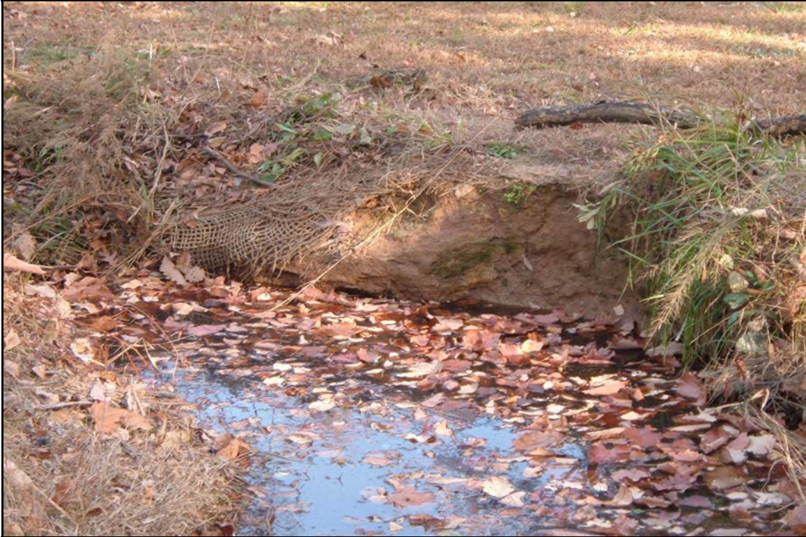
SP6 – Bank erosion. Photo taken near station 00+75. 11/5/06 - MY 02
