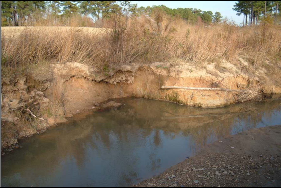
SP1 – Bank erosion. Photo taken near station 18+75. 11/5/06 - MY 02
