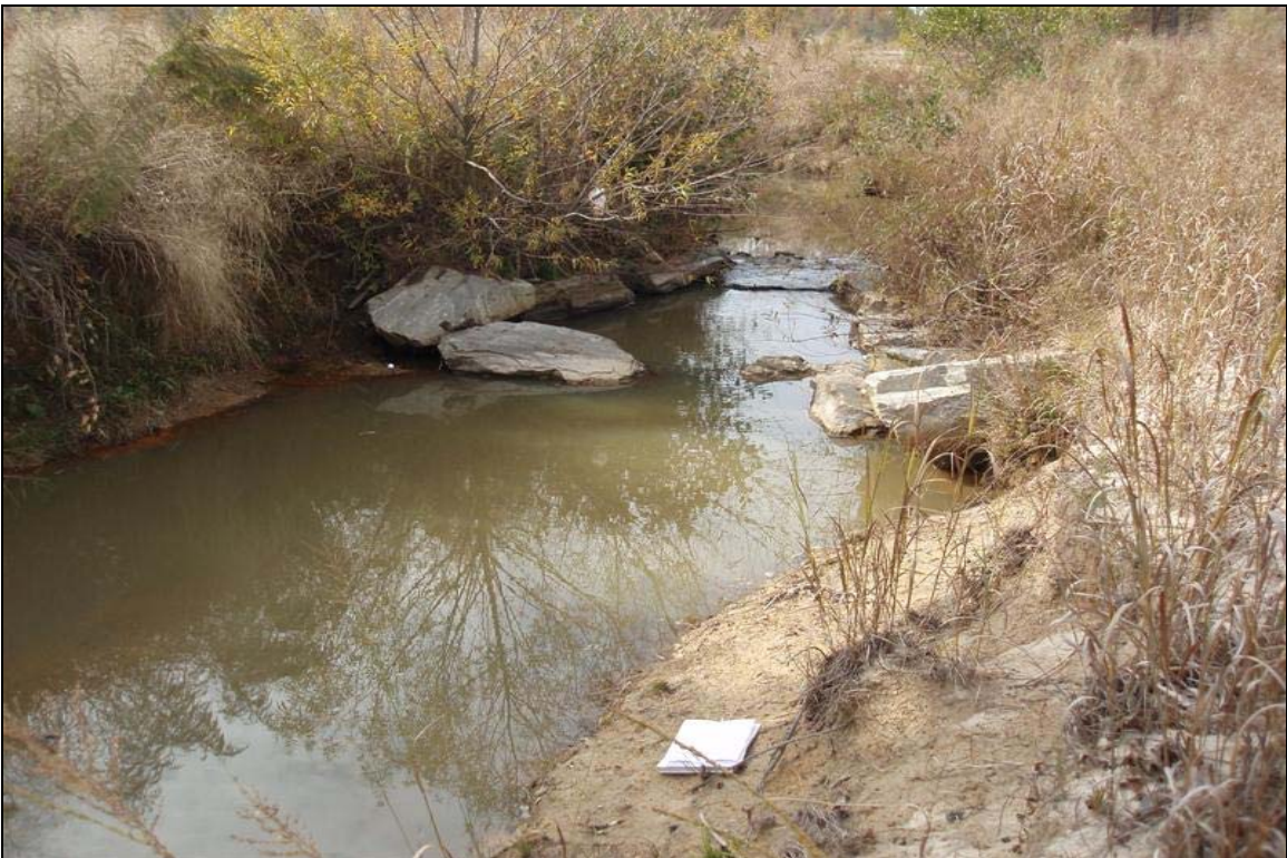
SP4 - Rock from cross vane has moved and bank has eroded behind cross vane arm. Photo taken near Station 16+75. 11/13/07 - MY 03
