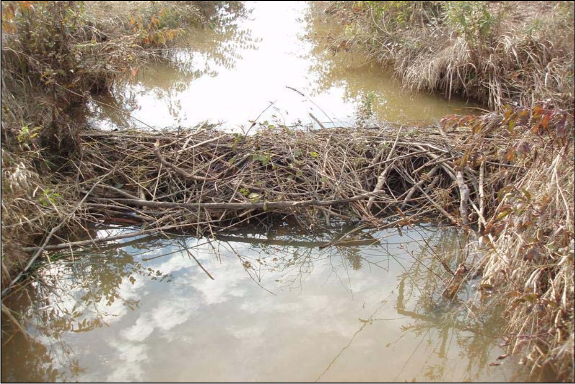
SP5 – Upstream Beaver dam. Photo taken near Station 49+75. 11/13/06 - MY 03
