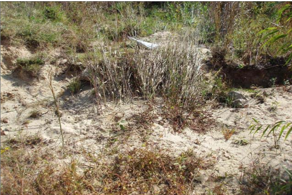
SP2 - Floodplain scour. Photo taken near Station 14+75. 10/27/08 - MY 04.
