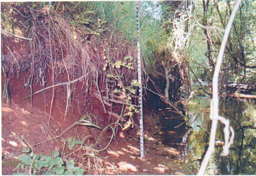
Picture 3. Undercut banks with no vegetation.
