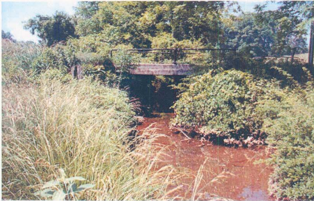
Picture 10. One-lane bridge looking upstream.
