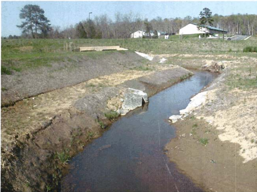
M16-DS: View from Meander 16 looking downstream. Cross-vane is drowned out due to backwater from the off-site lake downstream.
