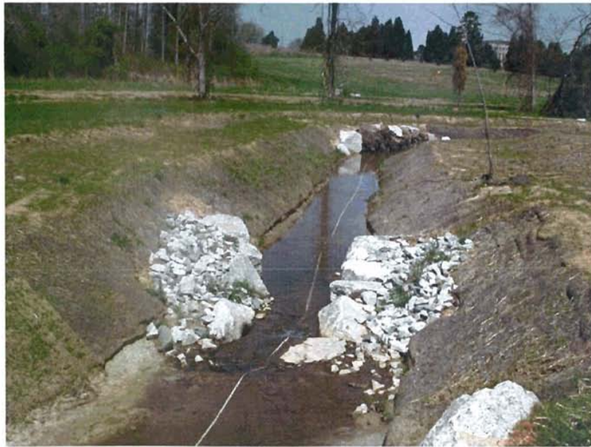
M4-DS: View from Meander 4 looking downstream towards Meander 5.
