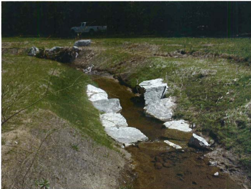
M3-DS: View from Meander 3 looking downstream towards a cross vane that was installed after the main construction period due to concerns with the grade downstream.
