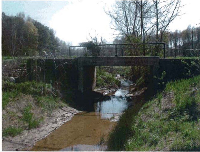
M12-US: View from Meander 12 looking upstream through the culvert.
