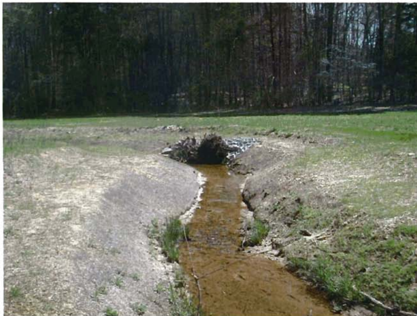
MI-DS: View from Meander 1, looking downstream towards M2.
