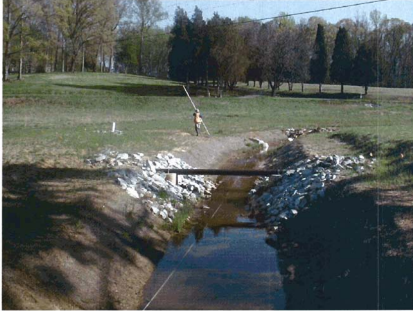
M16-US: View from Meander 16 looking upstream. The aerial sewer line was re-routed to make it perpendicular to the stream.
