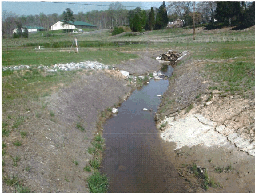
M14-DS: View from Meander 14 looking downstream. Note stone step-pool outfall to connect roadway drainage to stream.
