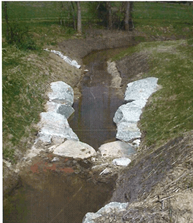
M6-DS: View from Meander 6 looking downstream. Note newly constructed cross-vane due to upstream degradation since the initial construction. Water is short cutting between the cross boulders on the right side.
