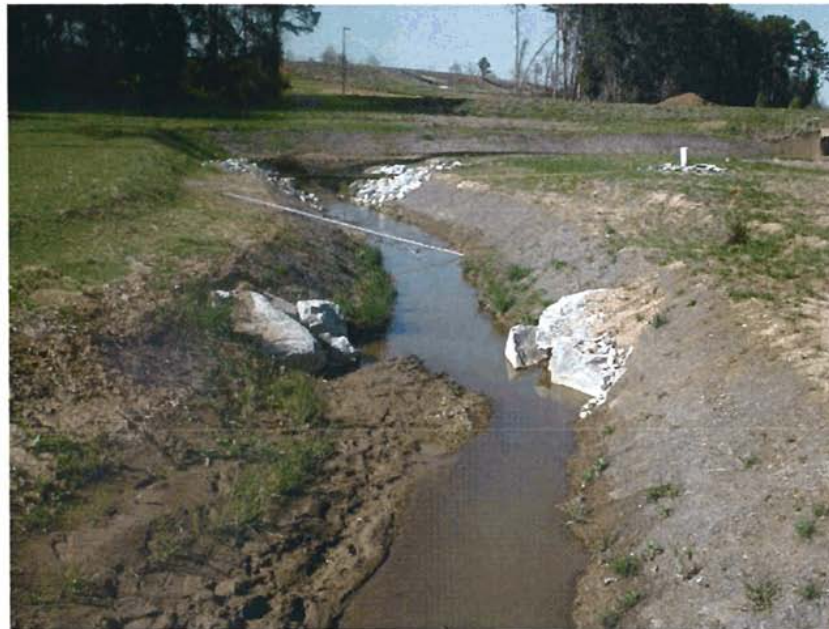
M15-DS: View from Meander 15 looking downstream. Note this cross-vane was moved upstream into the meander to avoid a gas line during construction. In effect, the upper portion of the cross vane has been covered up by the point bar since the cross vane slowed the water on the inside meander.
