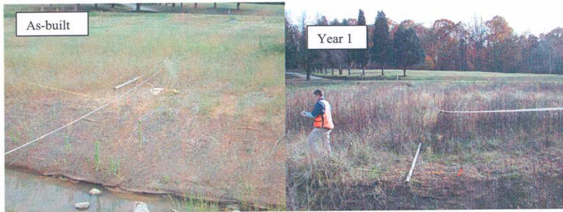
Transect 9 (BT9-R) – View of right bank, build-out bench and buffer.
