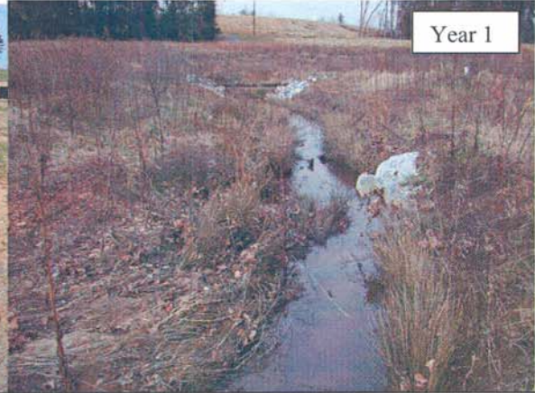
M15-DS: View from Meander 15 looking downstream. Note this cross-vane was moved upstream into the meander to avoid a gas line during construction. In effect, the upper portion of the cross vane has been covered up by the point bar.
