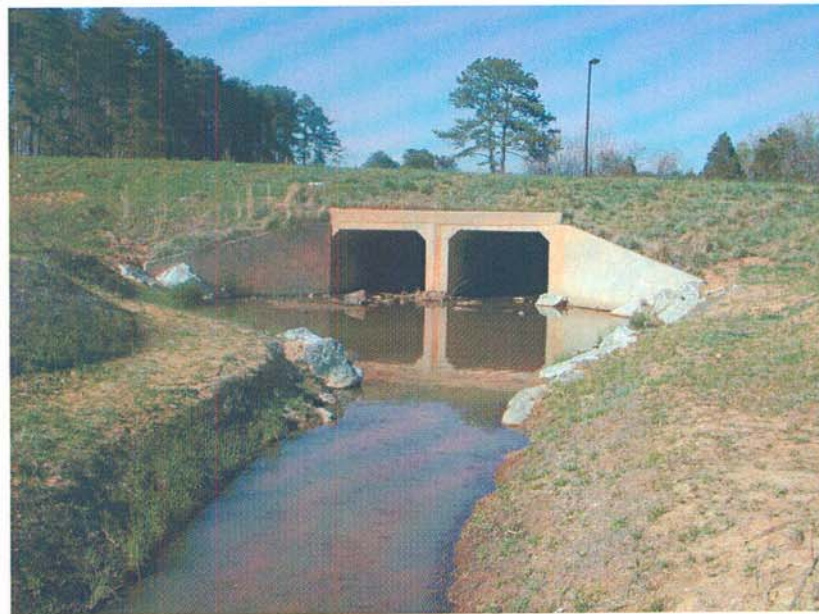
M17-DS: View from Meander 17 looking downstream towards the double 10' x 8' box culvert. Cross-vane is drowned out.
