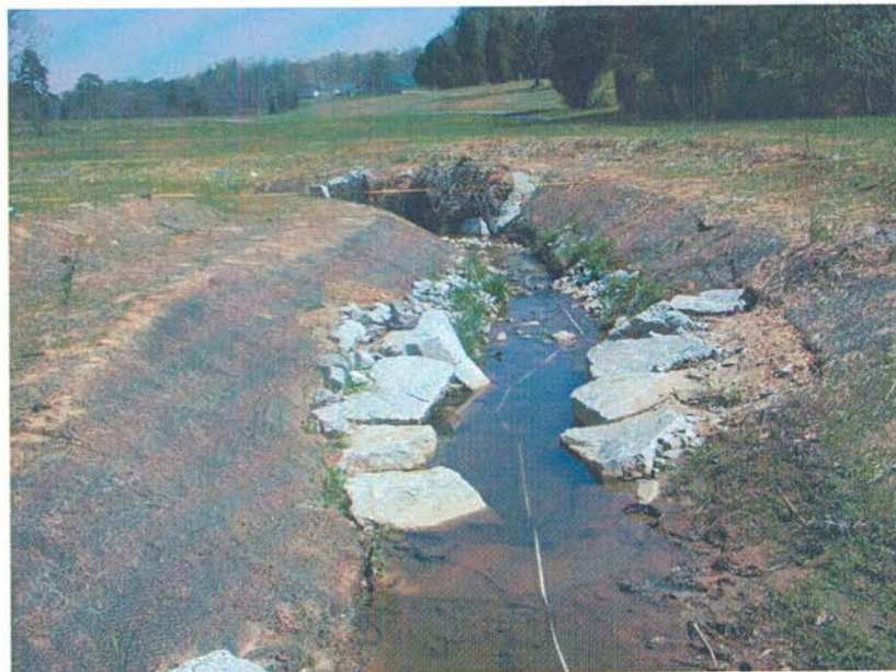
M5-DS: View from Meander 5 looking downstream towards Meander 6. Note the cross rock and the boulder adjacent to it on the right have settled since construction and are below the water surface.
