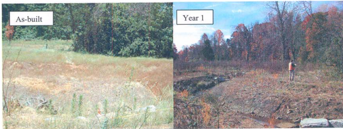
Transect 4 (BT4-L)– Left bank. Looking at area disturbed by construction of new structure.
