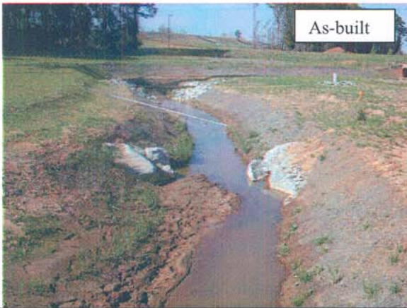
M15-DS: View from Meander 15 looking downstream. Note this cross-vane was moved upstream into the meander to avoid a gas line during construction. In effect, the upper portion of the cross vane has been covered up by the point bar.
