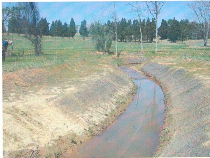
M8-DS: View from Meander 8 looking downstream towards Meander 9. Meander 9 does not have rootwads since the existing trees were salvaged.
