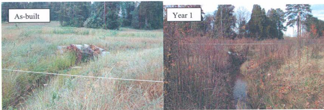
Transect 8 (BT8-D)– Right build-out bench looking downstream. Shows relatively dense herbaceous vegetation.
