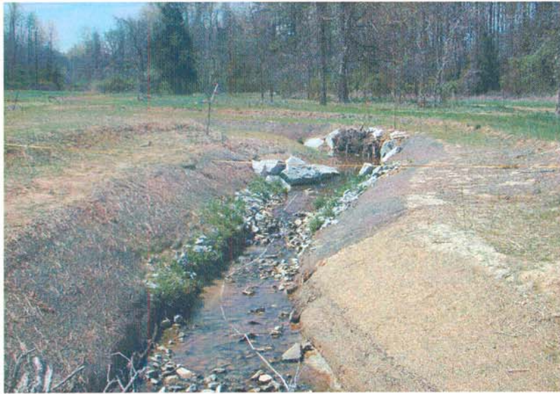
M6-US: View from Meander 6 looking upstream towards Meander 5. Note rip-rap was installed at the end of construction due to bed downcutting.
