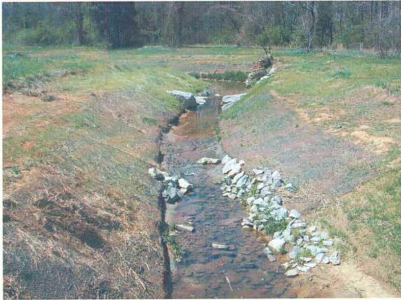
M4-US: View from Meander 4 looking upstream at Meander 3.
