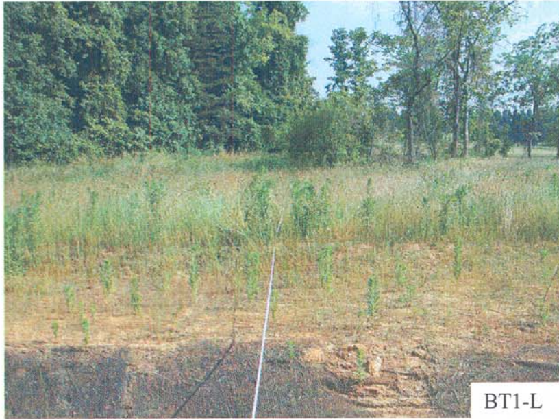
Transect 1 – Left bank. Shows build-out bench above coir matting with thin herbaceous vegetation
