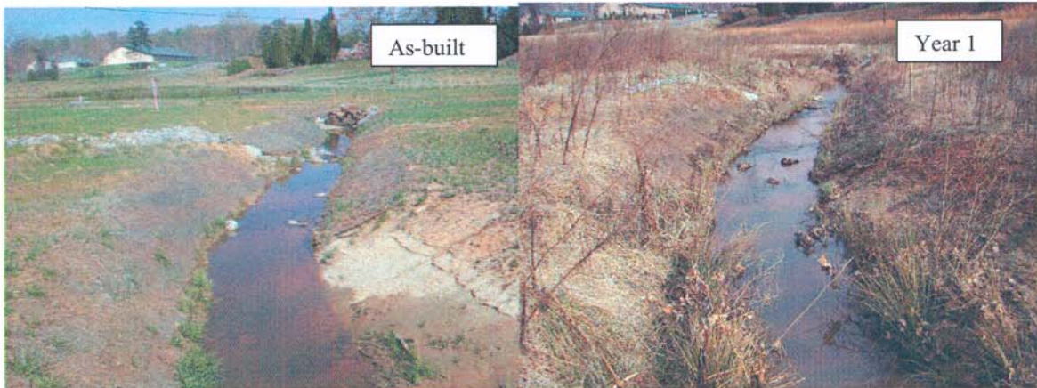
M14-DS: View from Meander 14 looking downstream. Note stone step-pool outfall to connecting roadway drainage to stream channel.
