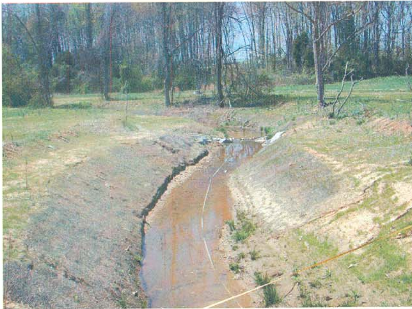
M8-US: View from Meander 8 looking upstream. Note the yellow fiberglass tape is pulled across the pool cross section in the foreground.
