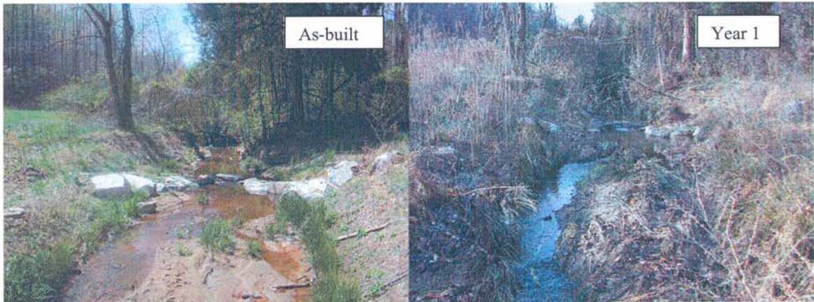
M1-US: Meander 1, looking in the upstream direction. Fenceline represents the beginning of the project and longitudinal profile. Note bar formation and vegetation establishment in this region.
