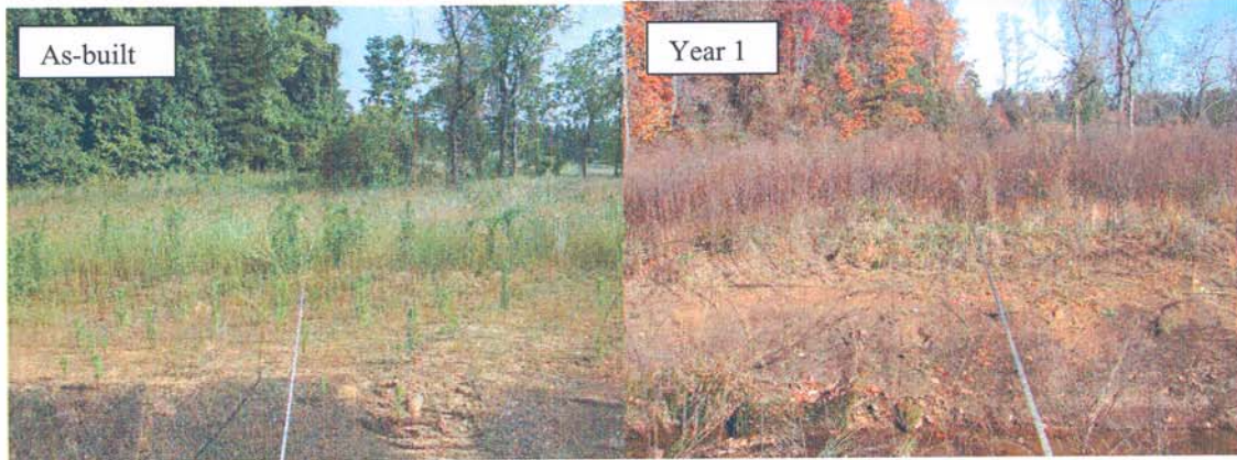
Transect 1 (BT1-L) – Left bank. Shows build-out bench above coir matting with thin herbaceous vegetation
