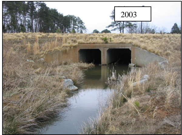
M17-DS: View from Meander 17 looking downstream towards the double 10' x 8' box culvert. Cross-vane is drowned out.88
