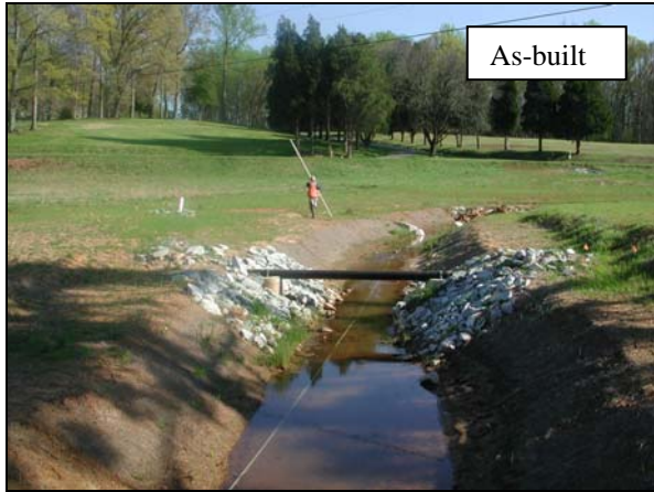
M16-US: View from Meander 16 looking upstream. The aerial sewer line was re-routed to make it perpendicular to the stream. 85
