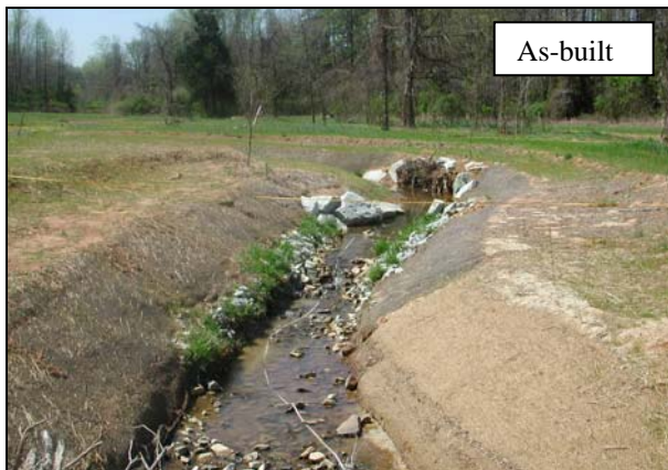
M6-US: View from Meander 6 looking upstream towards Meander 5. Note rip-rap was installed at the end of construction due to bed downcutting. 64
