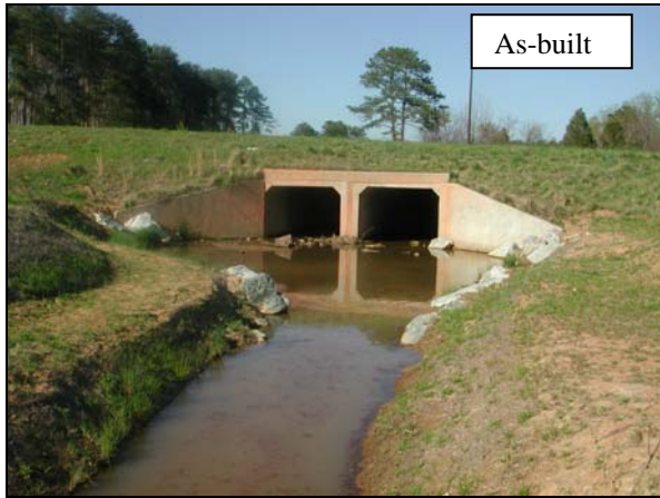
M17-DS: View from Meander 17 looking downstream towards the double 10' x 8' box culvert. Cross-vane is drowned out.88
