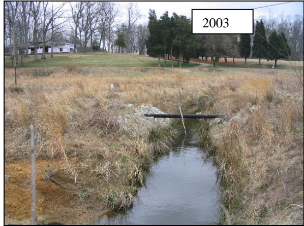
M16-US: View from Meander 16 looking upstream. The aerial sewer line was re-routed to make it perpendicular to the stream. 85
