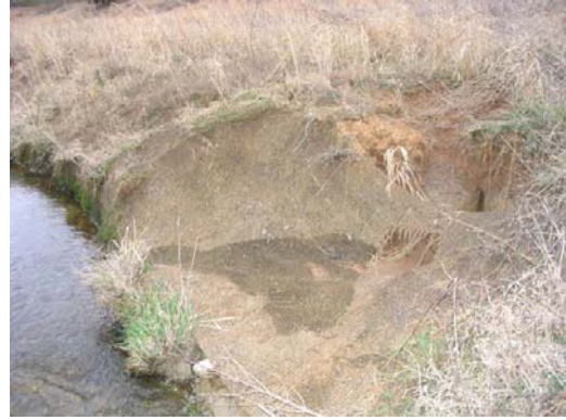
Issue Photo 12 – Station 13+60 Overland flow eroding channel bank
