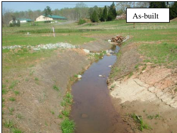
M14-DS: View from Meander 14 looking downstream. Note stone step-pool outfall to connecting roadway drainage to stream channel.82
