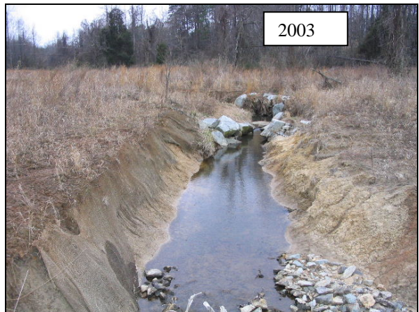
M6-US: View from Meander 6 looking upstream towards Meander 5. Note rip-rap was installed at the end of construction due to bed downcutting. 64
