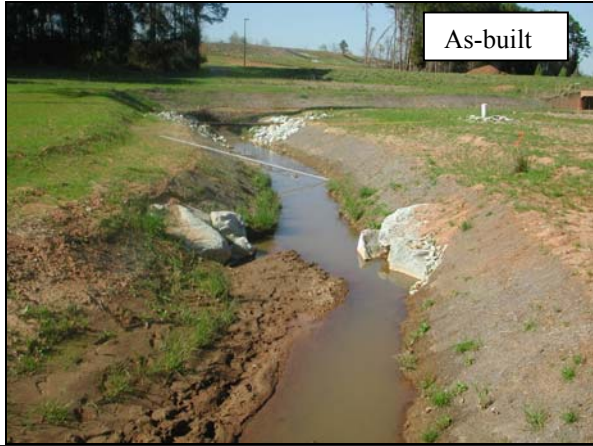
M15-DS: View from Meander 15 looking downstream. Note this cross-vane was moved upstream into the meander to avoid a gas line during construction. In effect, the upper portion of the cross vane has been covered up by the point bar. 84
