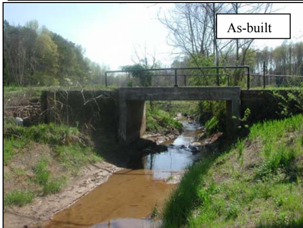
M11-DS: View from Meander 11 looking downstream. Jefferson Club Road crosses the stream via this 14' x 7.5 box culvert. 75
