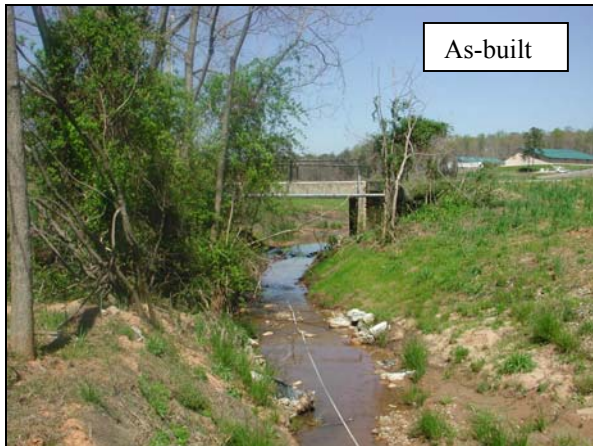
M11-DS: View from Meander 11 looking downstream. Jefferson Club Road crosses the stream via this 14' x 7.5 box culvert. 75
