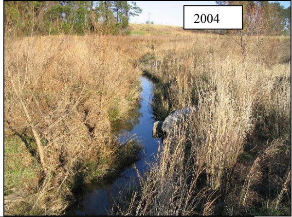
M15-DS: View from Meander 15 looking downstream. Note this cross-vane was moved upstream into the meander to avoid a gas line during construction. In effect, the upper portion of the cross vane has been covered up by the point bar. 84
