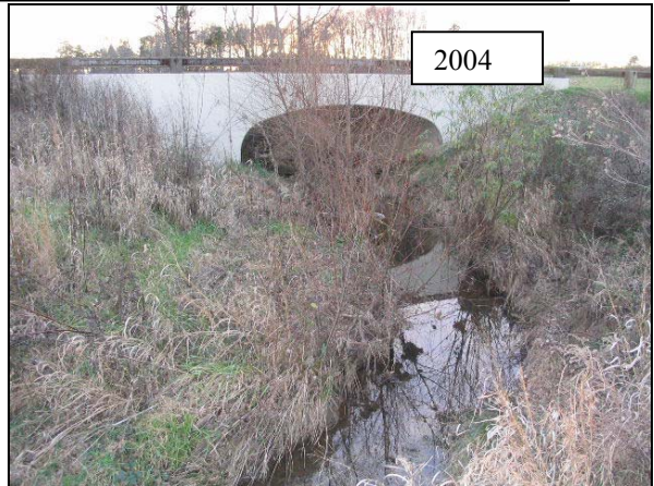
M11-DS: View from Meander 11 looking downstream. Jefferson Club Road crosses the stream via this 14' x 7.5 box culvert. 75
