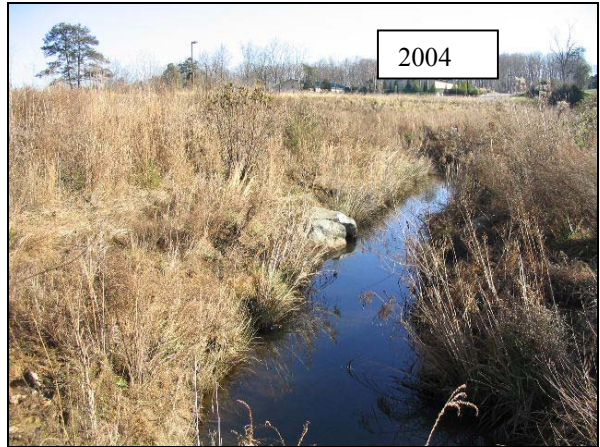
M16-DS: View from Meander 16 looking downstream. Cross-vane is drowned out due to backwater from the off-site lake downstream. 86
