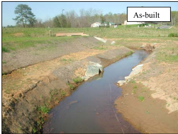
M16-DS: View from Meander 16 looking downstream. Cross-vane is drowned out due to backwater from the off-site lake downstream. 86
