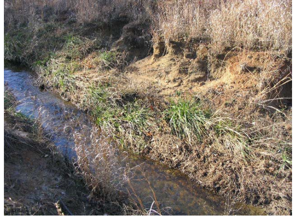
Issue Photo 8 - Station 4+40 Overland flow eroding channel bank
