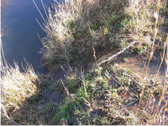
Issue Photo 13 - Station 16+20. Concentrated flow leaving wetland. Scouring streambank.
