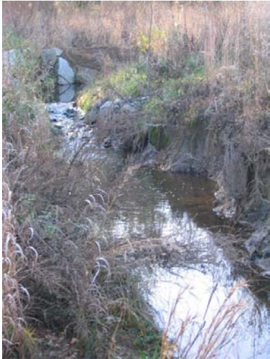
Issue Photo 3 - Station 1+50 Vertical and un-vegetated left bank
