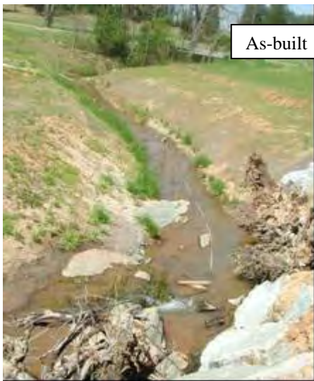
P20: View from Meander 10 looking downstream. Note the bedrock in the bed of the channel exposed during construction.73
