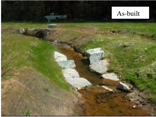
P6: View from Meander 3 looking downstream towards a cross vane that was installed after the main construction period due to concerns with the grade downstream.
