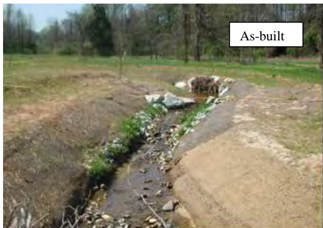
P11: View from Meander 6 looking upstream towards Meander 5. Note rip-rap was installed at the end of construction due to bed downcutting. 64
