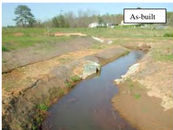
P32: View from Meander 16 looking downstream. Cross-vane is drowned out due to backwater from the off-site lake downstream. 86
