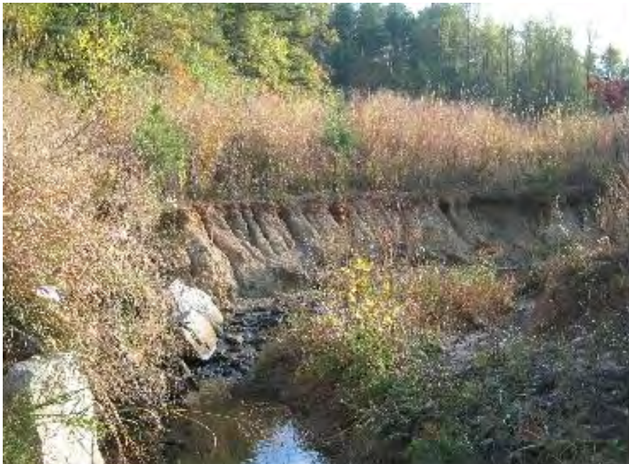
P9. Bank Erosion
