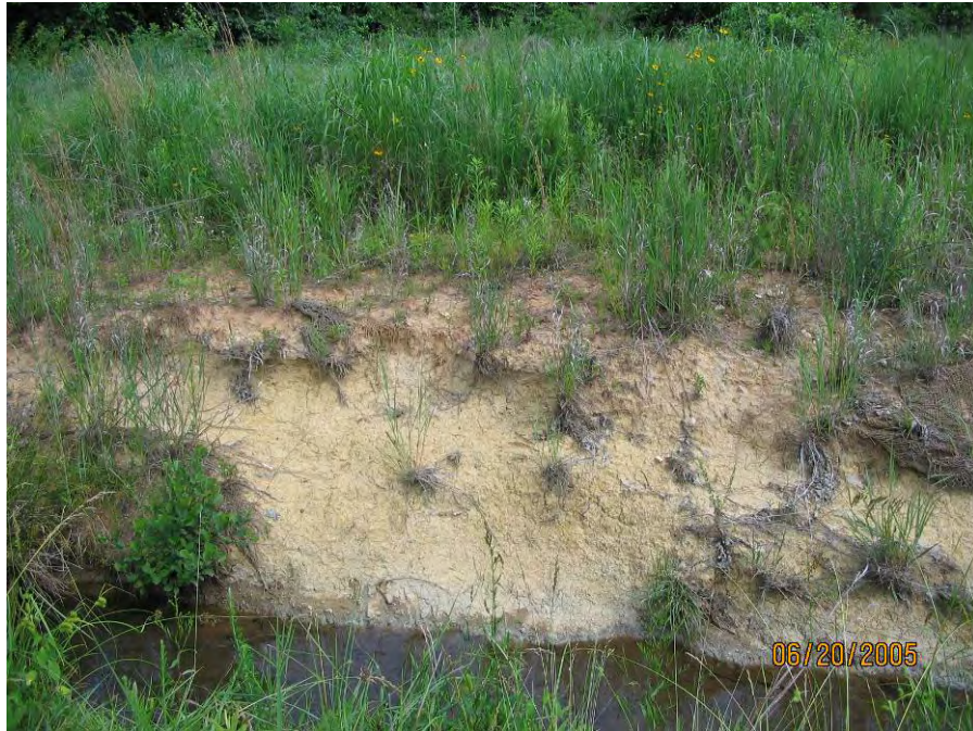
P1a. Bank Erosion
