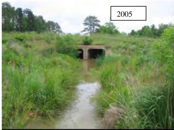
P34: View from Meander 17 looking downstream towards the double 10' x 8' box culvert. Cross-vane is drowned out.88
