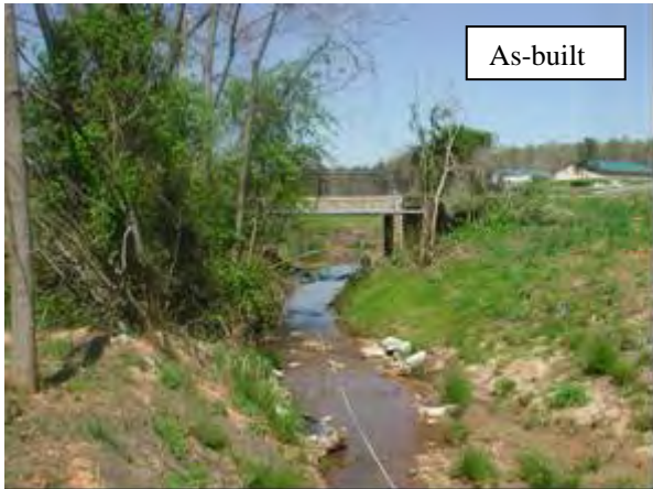
P22: View from Meander 11 looking downstream. Jefferson Club Road crosses the stream via this 14' x 7.5 box culvert. 75
