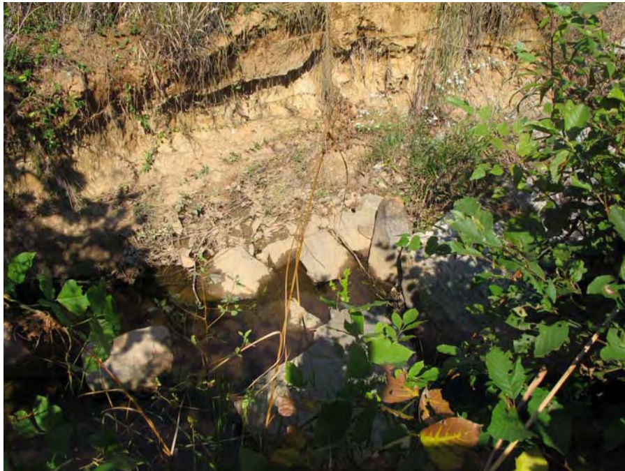
P13. Bank Erosion
