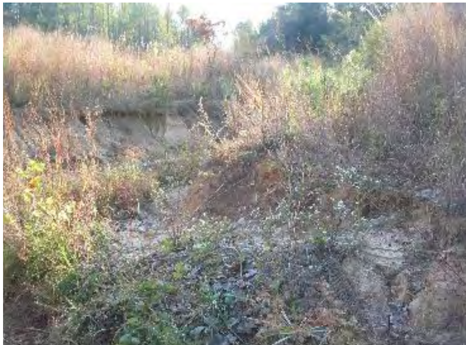
P14. Bank Erosion
