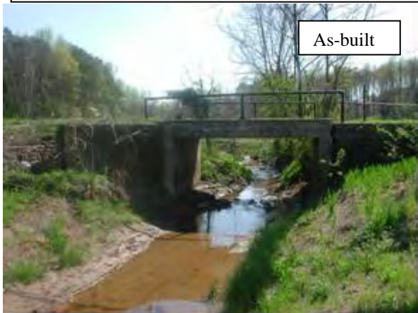
P22: View from Meander 11 looking downstream. Jefferson Club Road crosses the stream via this 14' x 7.5 box culvert. 75
