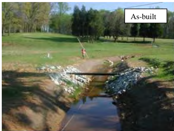
P31: View from Meander 16 looking upstream. The aerial sewer line was re-routed to make it perpendicular to the stream. 85
