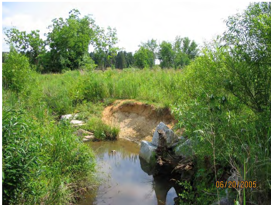
P5. Bank Erosion
