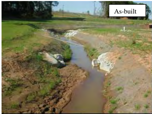
P30: View from Meander 15 looking downstream. Note this cross-vane was moved upstream into the meander to avoid a gas line during construction. In effect, the upper portion of the cross vane has been covered up by the point bar. 84
