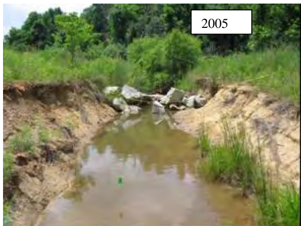
P11: View from Meander 6 looking upstream towards Meander 5. Note rip-rap was installed at the end of construction due to bed downcutting. 64
