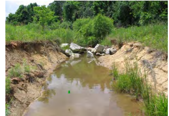
Photo of Cross-Section #1 - Looking Upstream
