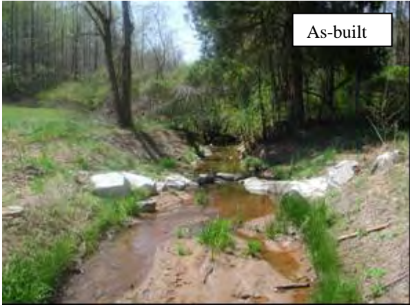
P1: Meander 1, looking in the upstream direction. Fenceline represents the beginning of the project and longitudinal profile. Note bar formation and vegetation establishment in this region.
