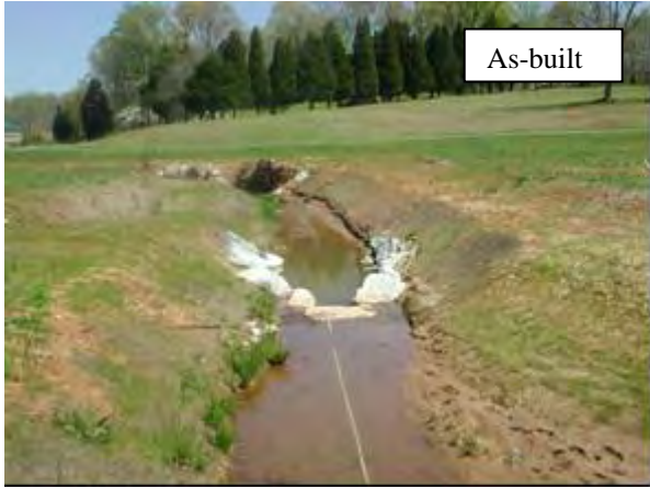
P18: View from Meander 9 looking downstream. Note the point bar formation in the lower right corner of picture.71
