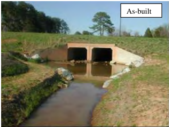
P34: View from Meander 17 looking downstream towards the double 10' x 8' box culvert. Cross-vane is drowned out.88
