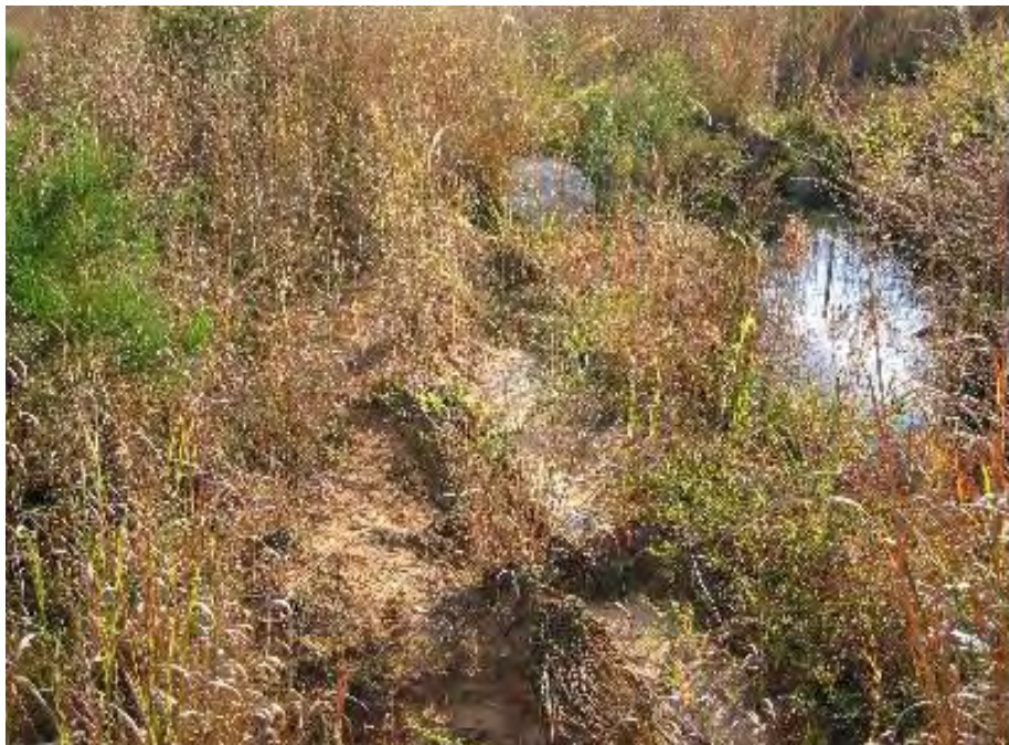
P16. Bank Erosion
