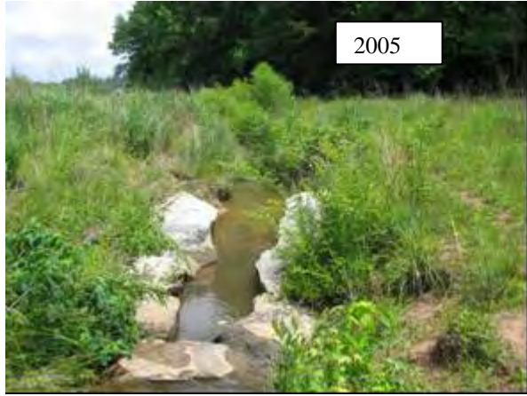
P6: View from Meander 3 looking downstream towards a cross vane that was installed after the main construction period due to concerns with the grade downstream.
