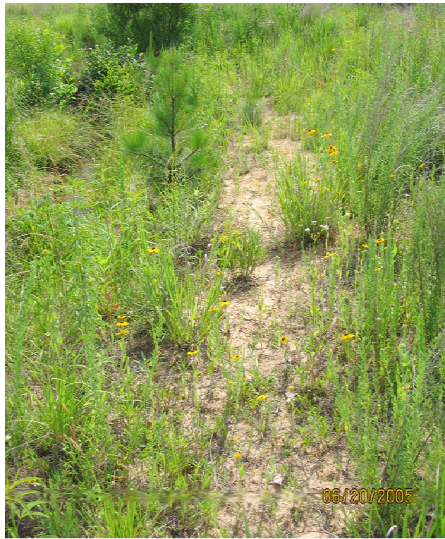
P12a. Bank Erosion
