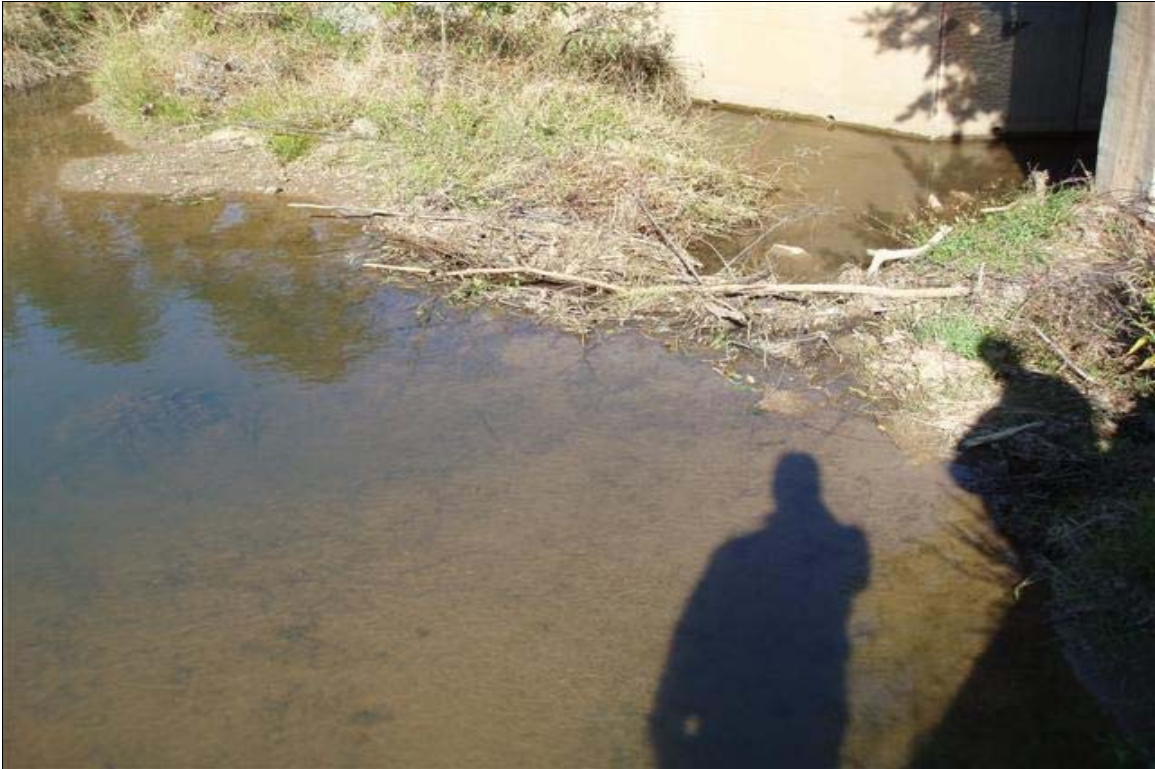
SP5 – Beaver dam causing backwater conditions to Station 13+60. Photo taken near Station 17+50. 10/29/08 - MY 06
