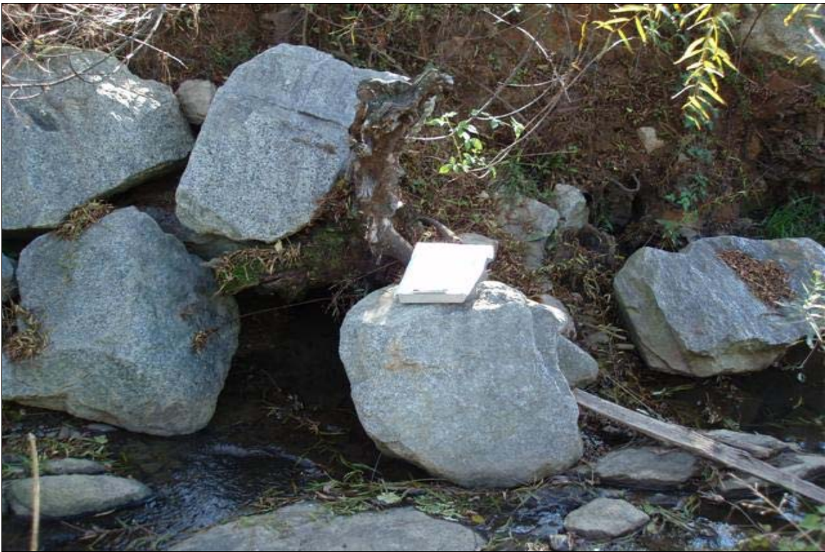
SP3 – Root wads completely above baseflow, rotting, and with scour behind. Photo taken near Station 9+00. 10/29/08 - MY 06
