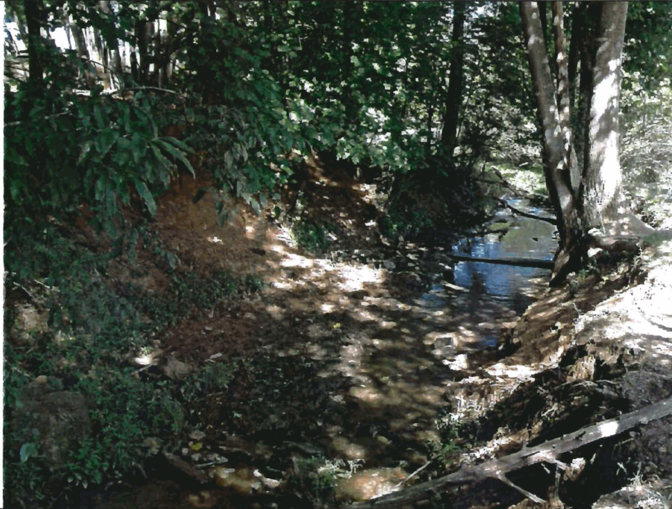
Photo 3: Looking upstream in channel 1a at eroding banks
