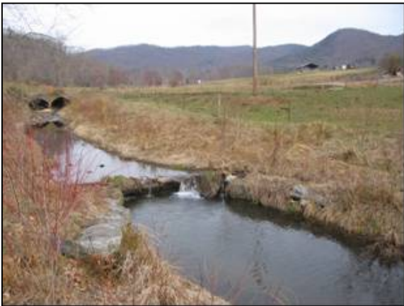
IP 22 Slump Arm and Piping (Below Study Reach)
