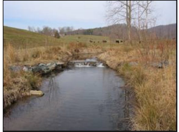
IP 40 Vane Undermine Rt. Arm (Station 3+50)
