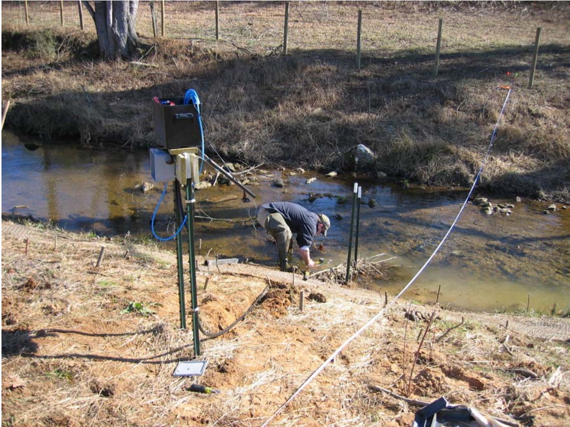
Figure 2: Installation of a Stage Monitoring and Grab Sample Station
