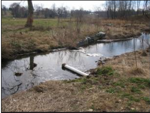
IP 39 Tile (Station 2+10)
