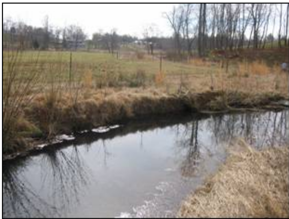
IP 41 Bank Erosion (Station 4+70)
