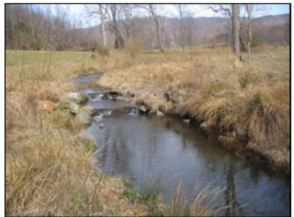
IP 17 Double Drop Vane w/ Erosion (Above Study Reach)
