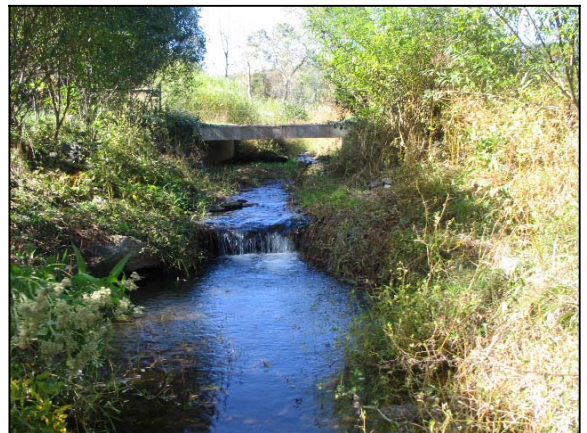
IP 8 Bed Elevation Drop Below Study Reach)
