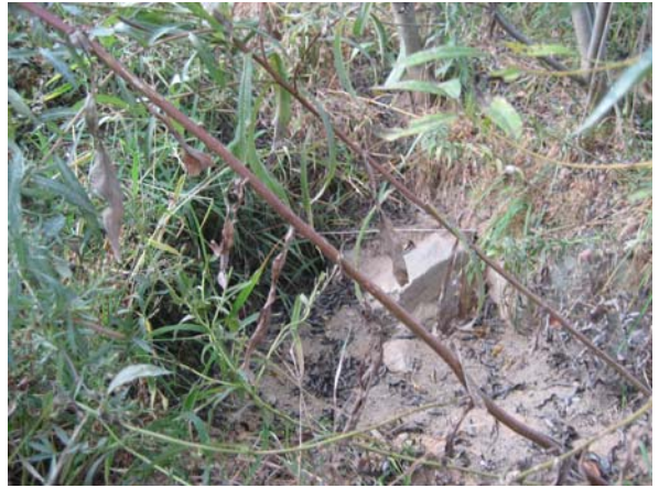
IP14a Piping through cross vane (Station 2+20) – Creek bed dry in 2007
