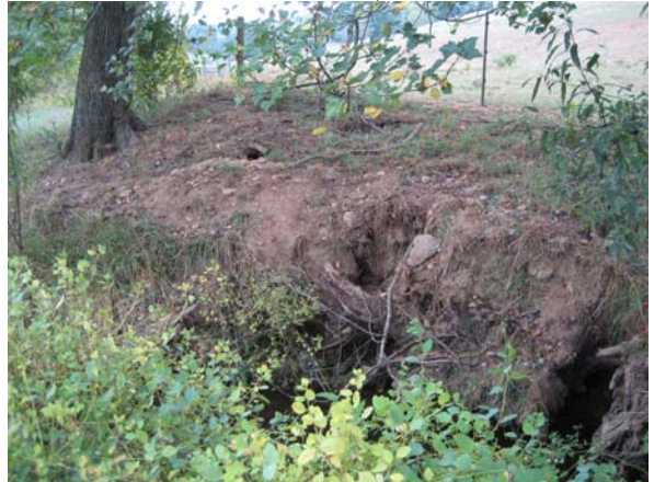
IP 20 Erosion Ground Hog Tunnels (Station 4+00)
