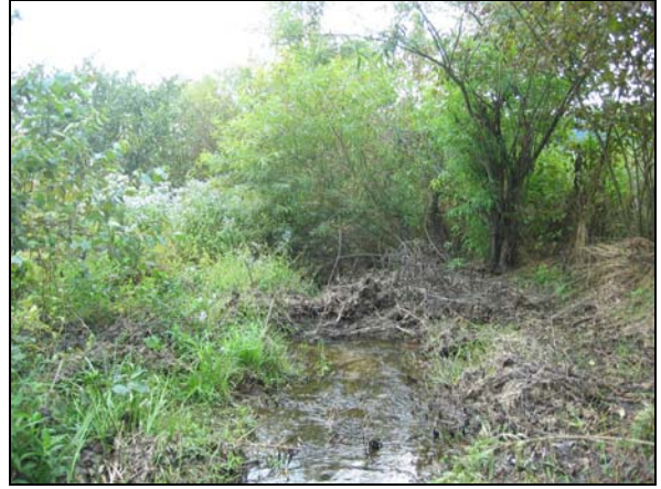
P37. X2 Downstream (Station 3+85)
