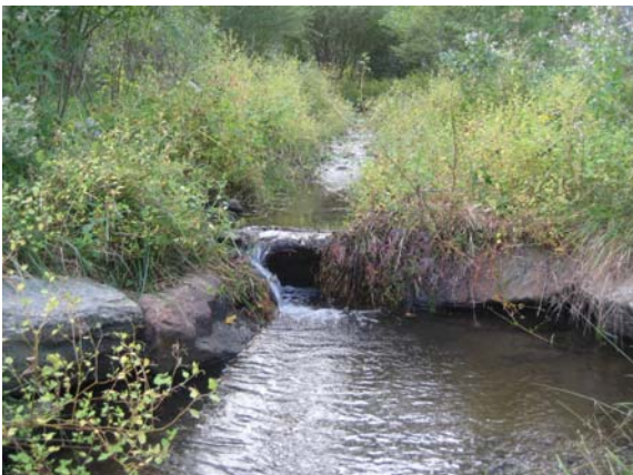
IP 5 Bed Elevation Drop and Piping at Left Arm (Station 0+89)
