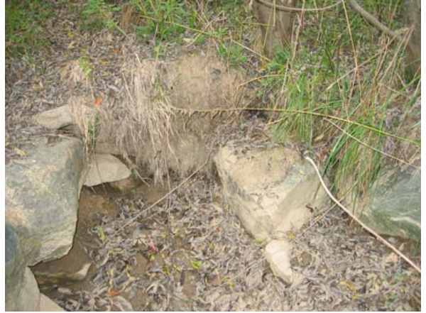
IP14a Piping through cross vane (Station 2+20) – Creek bed dry in 2007 and 2008
