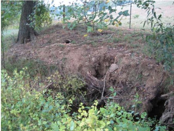
IP 20 Erosion Ground Hog Tunnels (Station 4+00)
