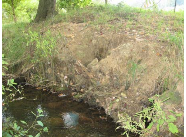
IP 20 Erosion Ground Hog Tunnels (Station 4+00)
