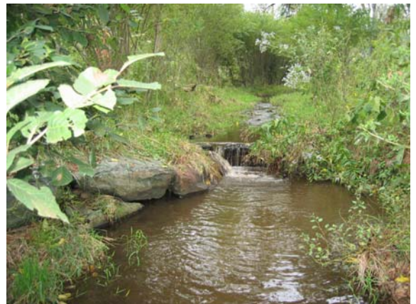
IP 7 Bed Elevation Drop (Station 5+50)
