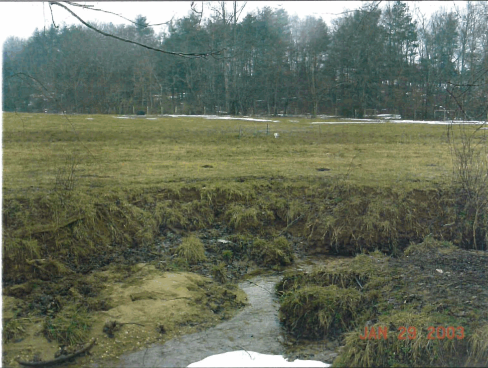
Photo 3: Downstream view of reach 4-(RDS-W2 in background). note downcutting and eroding banks
