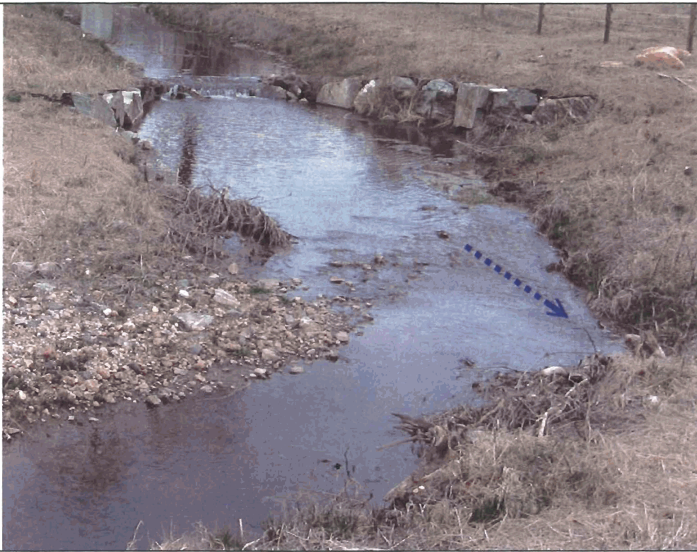
Photograph SP1 – Transverse bar directing flow into outside pool bank downstream..
