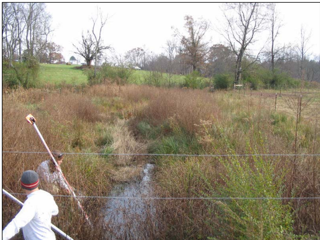
P26. Reach 4 – Bridge looking downstream
