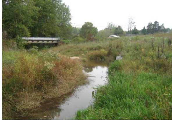
Photo of Cross-Section #10 - Looking Downstream
