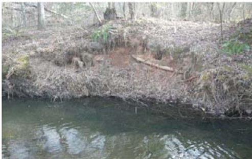
Photo 2. Bare area at Station 16+00 caused by past flooding, but appears stable at this time.
