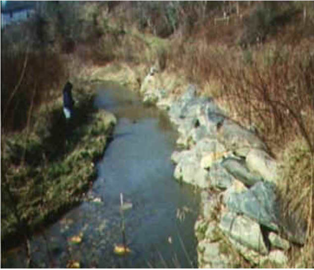
Existing riprap at stations 2+49 – 3+43 to be used to construct proposed rock vanes and cross vanes.
