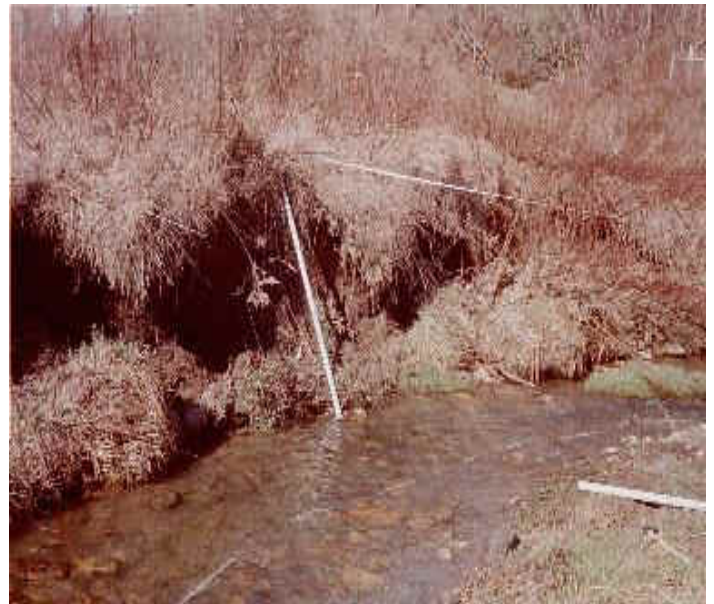
Eroding bank at station 1+86.
