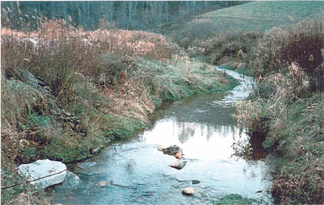
Looking upstream towards upper end of conservation easement. Laxon Creek before stream restoration work. This area contained a badly eroding bank and a riffle where a pool should have been. Banks were sloped and rock weirs installed to create a step/pool habitat. Location of cross-section 1+88.
