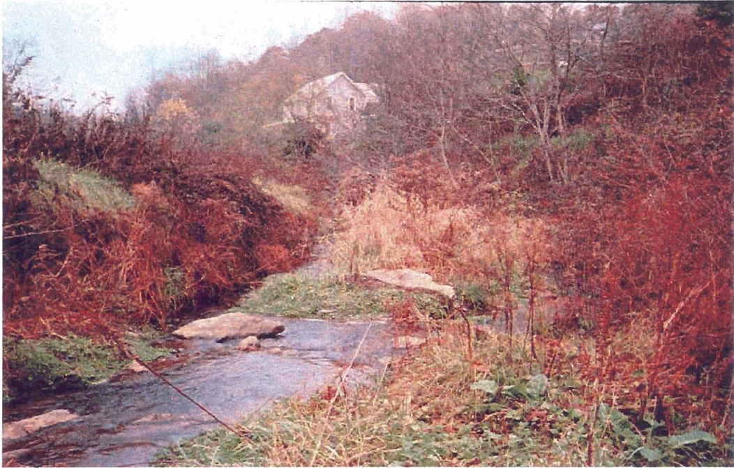
Braided channel and eroding left bank (looking downstream). Above: Before construction. Below: After construction showing bankfull bench, root wads and large boulders used to block off old channel and two rock weirs and one rock vane to create step/pool habitat and serve as grade controls. X-S 7+13
