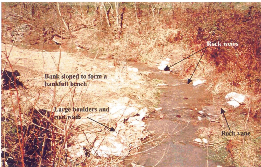
Braided channel and eroding left bank (looking downstream). Above: Before construction. Below: After construction showing bankfull bench, root wads and large boulders used to block off old channel and two rock weirs and one rock vane to create step/pool habitat and serve as grade controls. X-S 7+13
