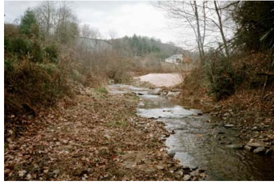
November 2, 2000 after construction.
