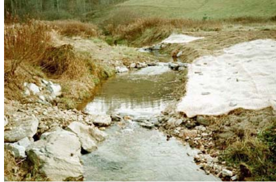
November 3, 2000 after construction.
