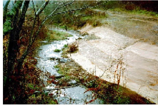
November 3, 2000 after construction.
