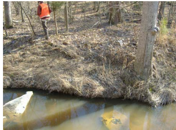
Photo 4: Representative undercut problem area (Station 30+82 along plan view).
