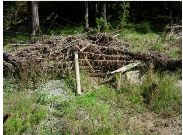
Photo 4: Representative cattle crossing fence damage problem area (Station No. 15+; view downstream on 10-13-2008). Note major damage to the fencing and debris caught in fencing above bankfull elevation (i.e. evidence of bankfull flow).
