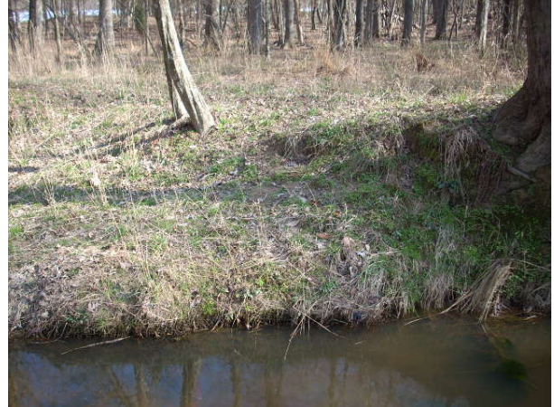
Photo 2: Representative undercut problem area (Station No. 23+41; view of right bank; 2-25-2008).
