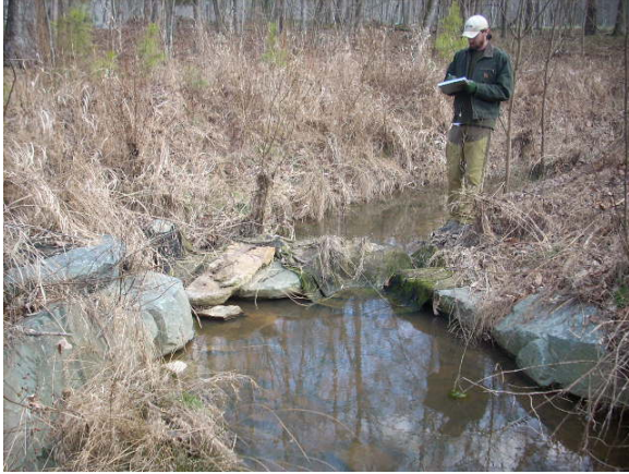
Photo 5: Representative problem crossvane (Station No. 32+86, view upstream on 2-25-2008).
