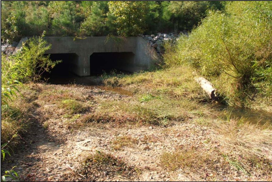
Photo Station 6 (Reach 2) – View looking upstream, towards culvert under Collector Rd.
