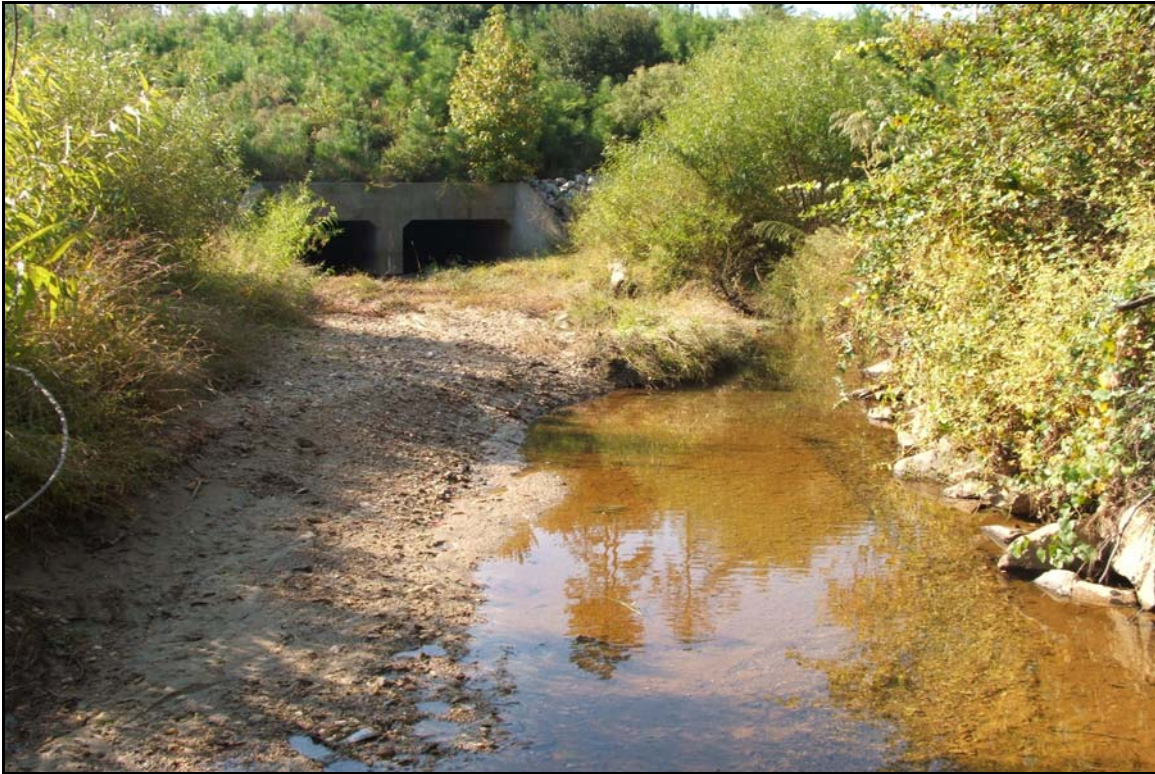
Photo Station 7 (Reach 2) – View looking upstream, towards culvert under Collector Rd.
