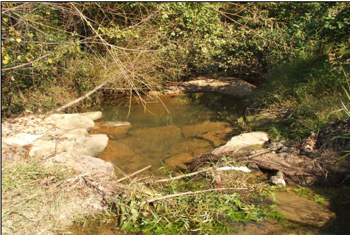
Photo Station 7 (Reach 2) – View looking downstream, with rock cross vane in foreground of photo.
