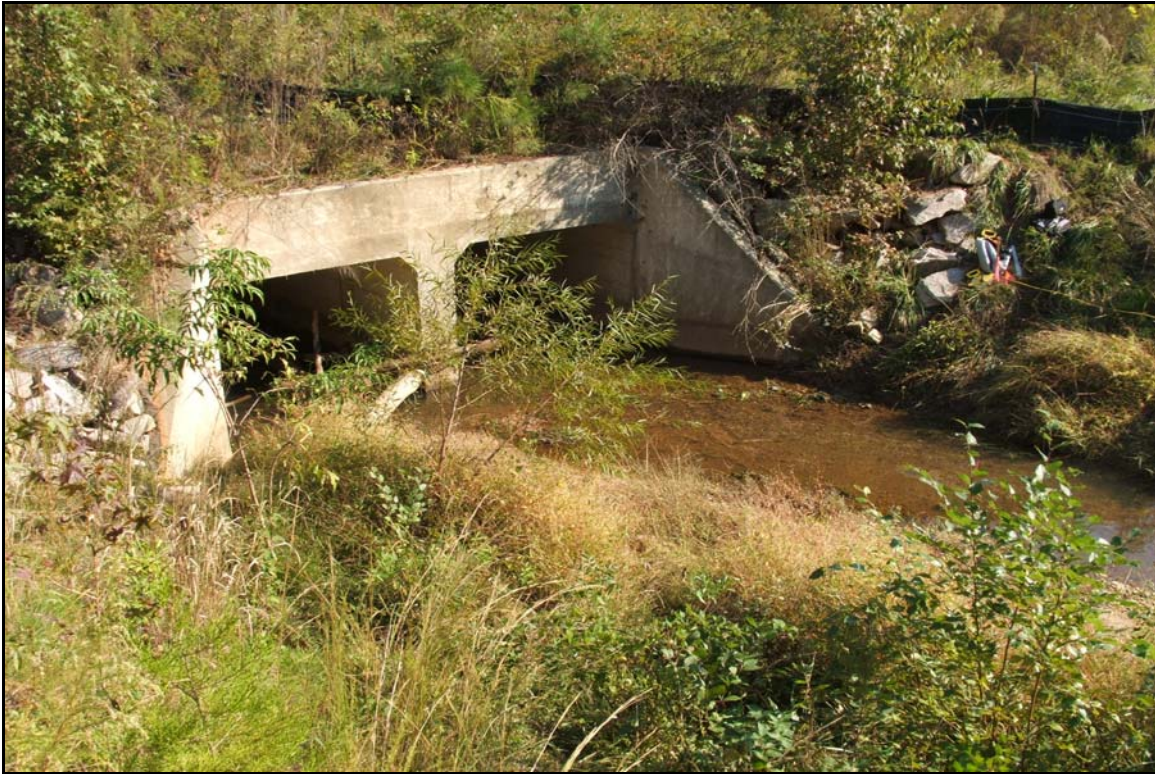
Photo Station 3 (Reach 1) – View looking northeast, towards culvert under Collector Rd.
