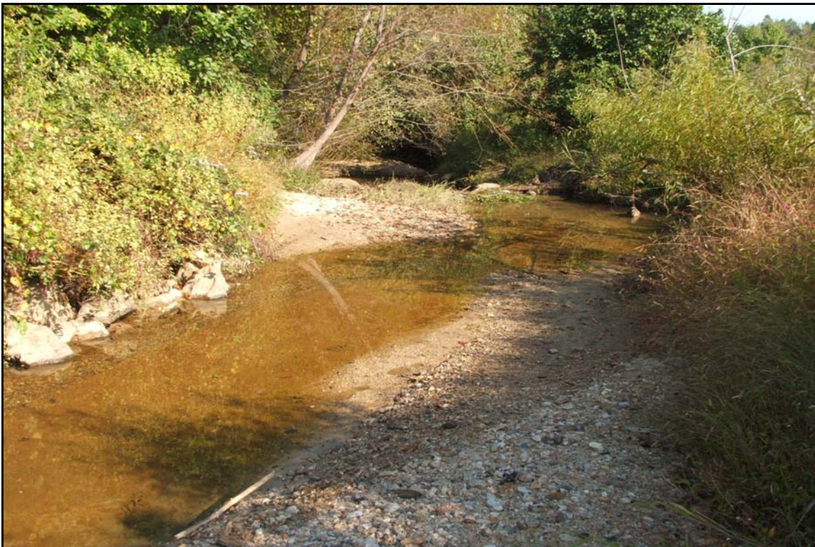
Photo Station 6 (Reach 2) – View looking downstream, towards rock cross vane.
