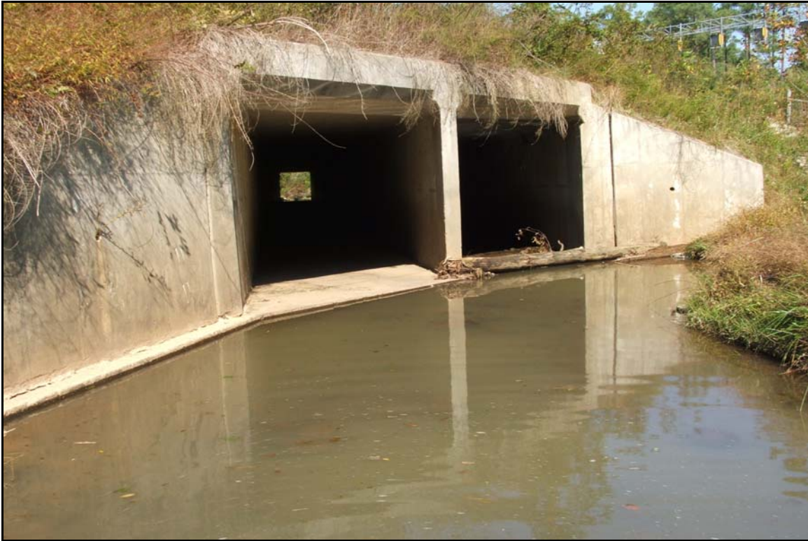
Photo Station 9 (Reach 3) – View looking downstream towards culvert under Edwards Mill Rd.
