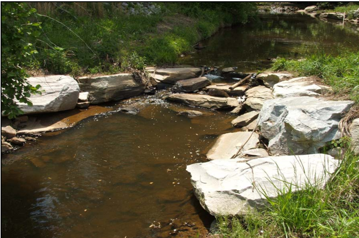
Photo Station 11 (Reach 3) – View looking upstream at rock cross vane.
