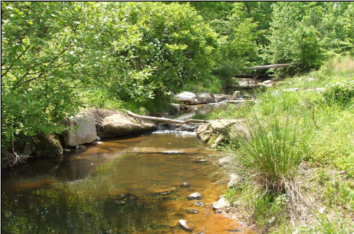
Photo Station 9 (Reach 3) – View looking upstream towards two rock cross vanes.
