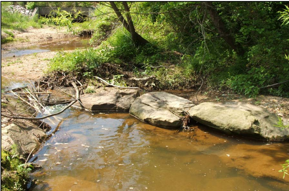
SP 2 (Reach 2) – Back arm scour on left arm of cross vane.
