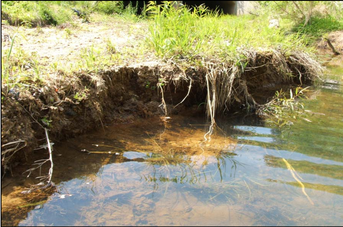
SP 1 (Reach 2) – Stream bank erosion on inside of upstream meander.
