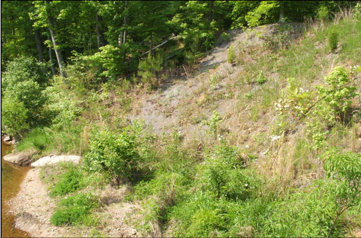
Photo Station 1 (Reach 1) – View looking southwest at the left bank and the slope above.
