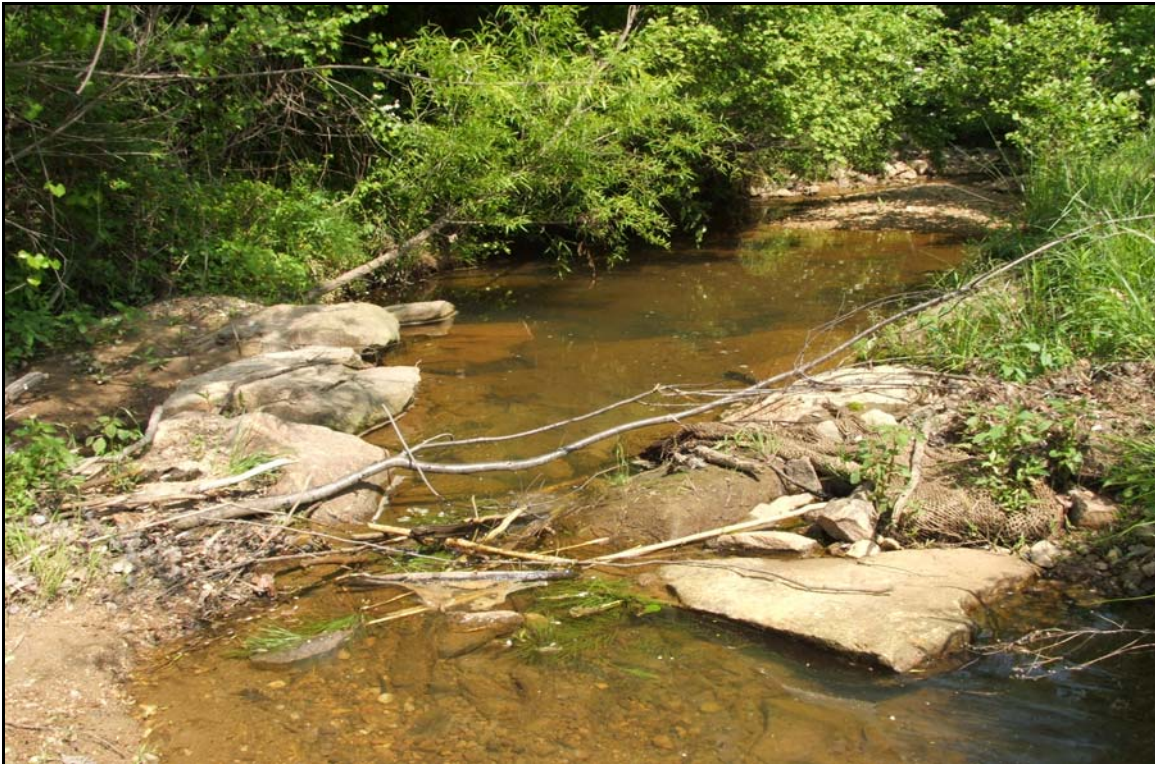
Photo Station 7 (Reach 2) – View looking downstream, with rock cross vane in foreground of photo.
