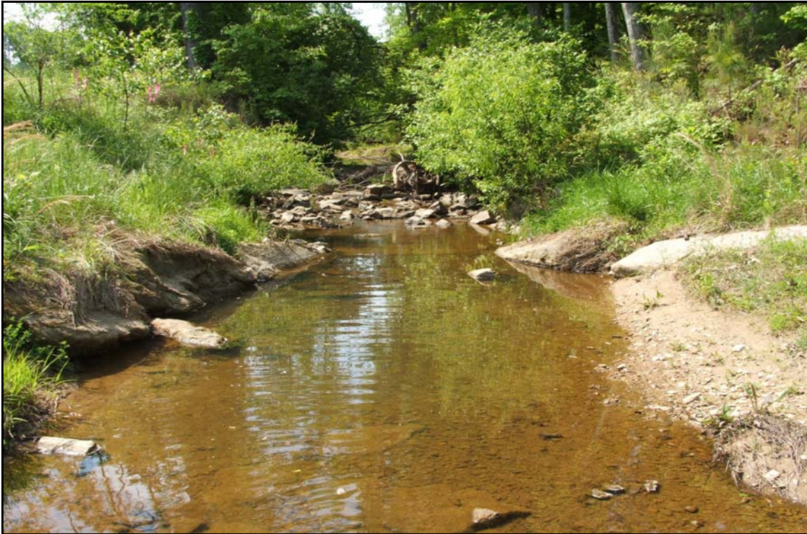
Photo Station 4 (Reach 1) – View looking upstream, with rock cross vane in center of photo.
