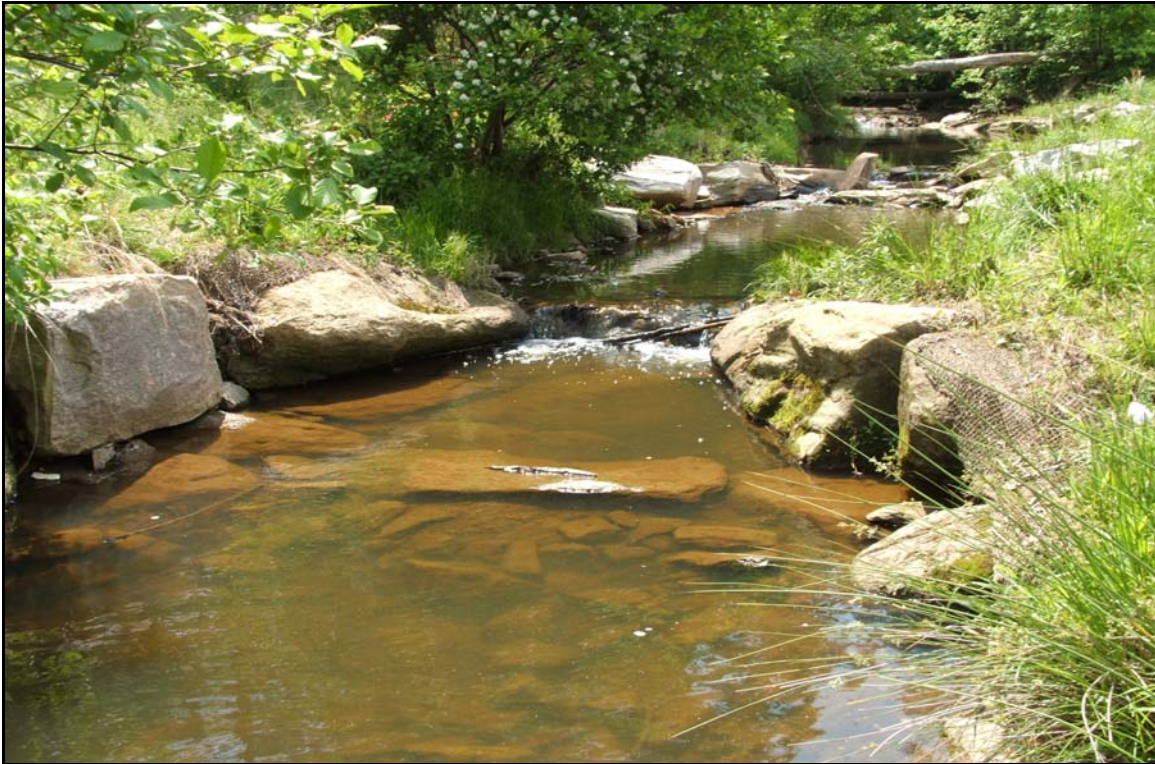
Photo Station 10 (Reach 3) – View looking upstream at rock cross vane.
