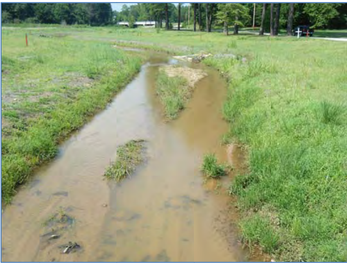
Photo Point #5 – Looking upstream from bridge 8/6/2010
