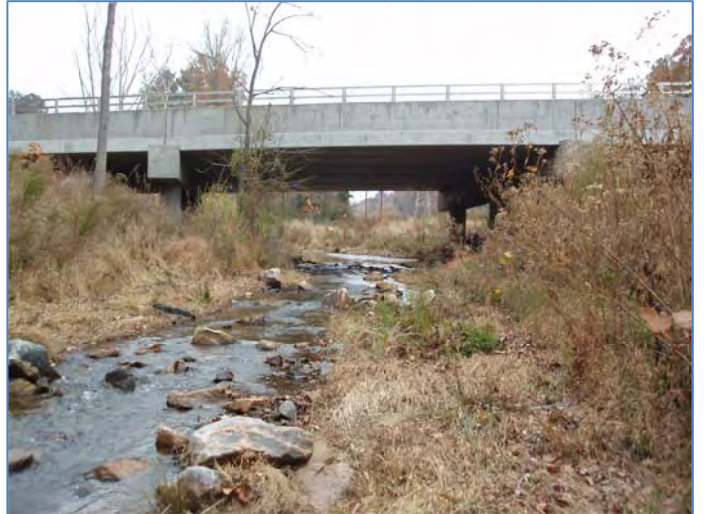
Photo Point #1 – Looking upstream at fish ramp 11/16/2011
