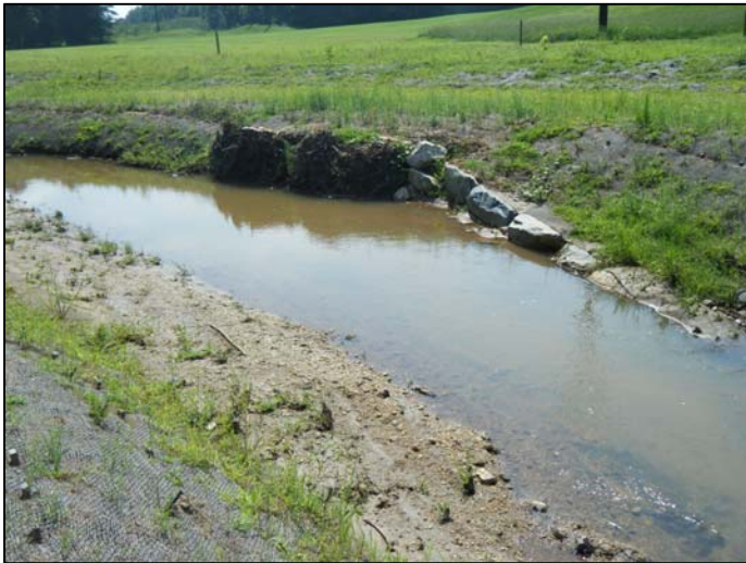
Photo Point #3 – Looking downstream 8/6/2010– Baseline
