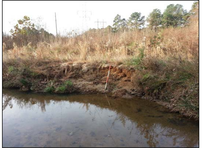
Station 4+00 Right Bank – 11/15/2013
