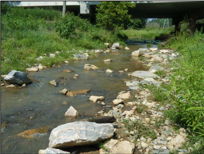
Photo Point #1 – Looking upstream at fish ramp 8/6/2010– Baseline
