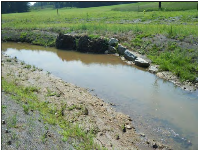
Photo Point #3 – Looking downstream 8/6/2010– Baseline
