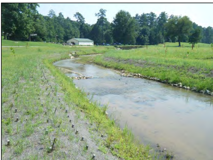
Photo Point #4 – Looking downstream 8/6/2010– Baseline
