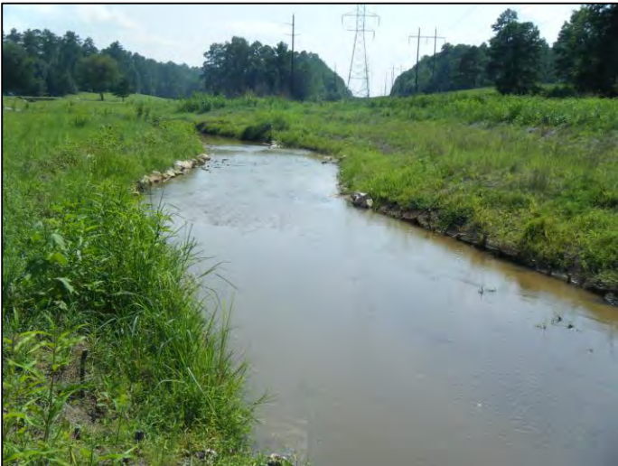
Photo Point #2 – Looking downstream 8/6/2010– Baseline
