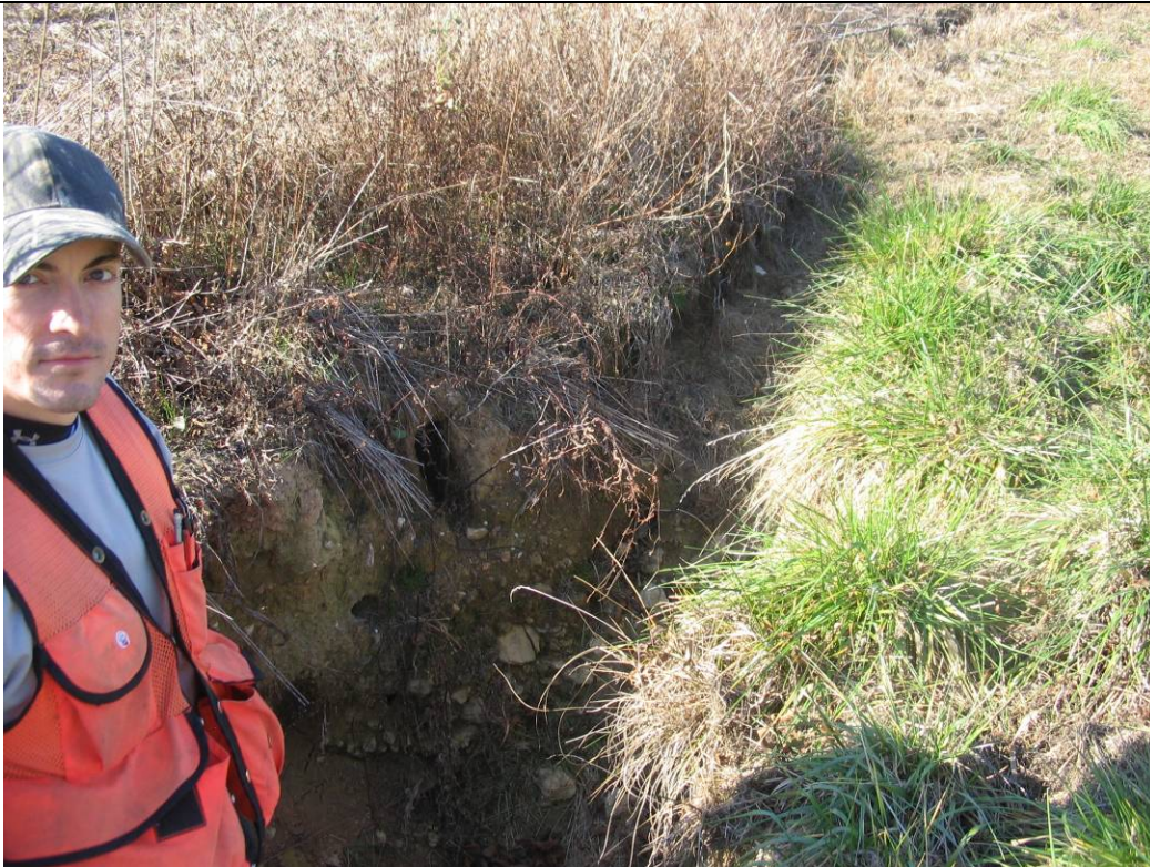
Photograph 11. Upper Reach of UT1.
