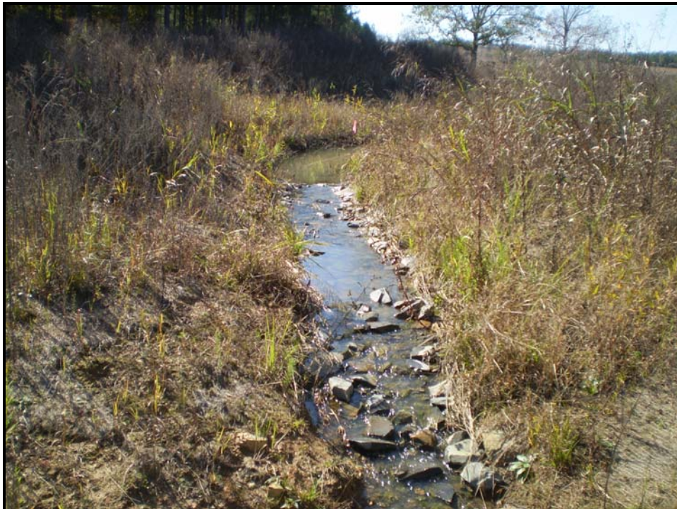
Stream Photo # 24 Constructed Riffle Looking Upstream at Sta. 443+45
