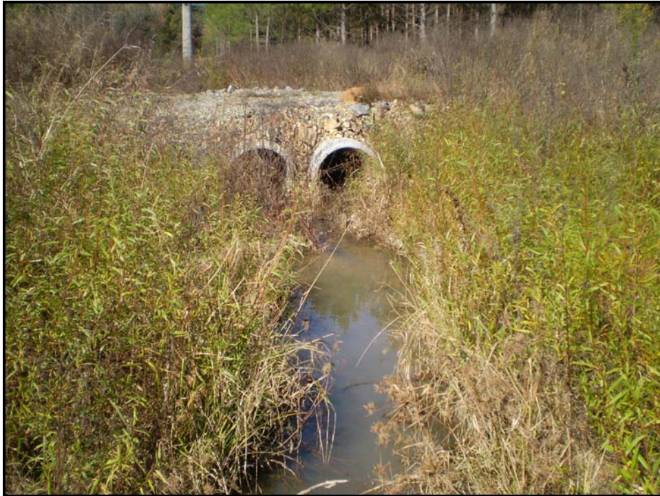
Stream Photo # 18 Upstream at Sta. 417+50
