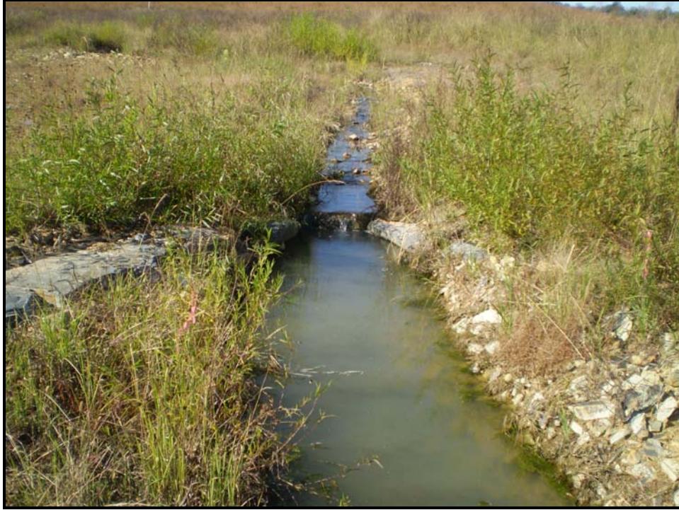
Stream Photo # 25 Rock Cross Vane Looking Upstream at Sta. 447+00
