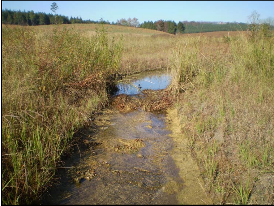
SPA # 1. Head cut with minor erosion at Sta. 138+75
