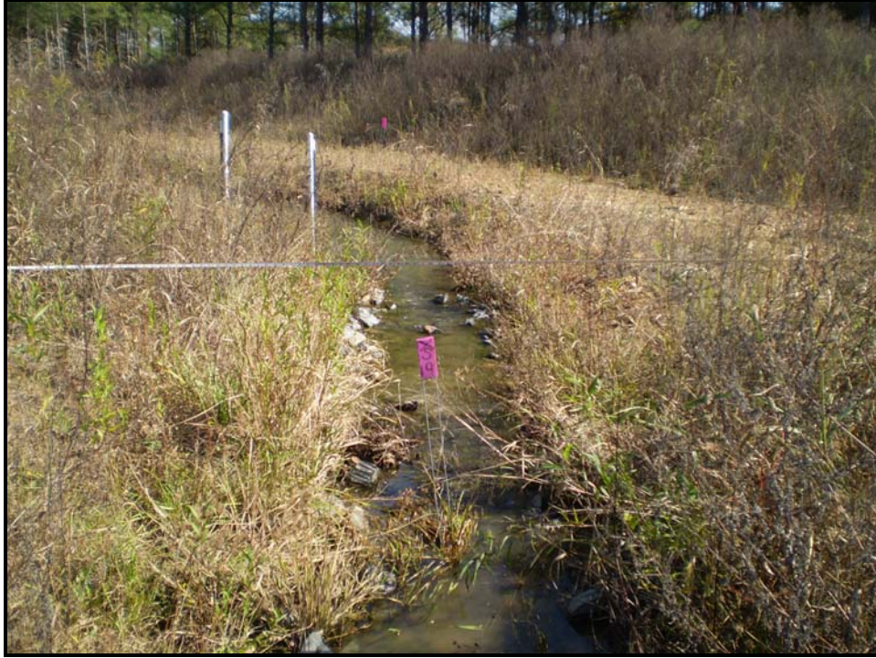
Stream Photo # 23 Looking Downstream at Cross-Section 19 Sta. 437+73
