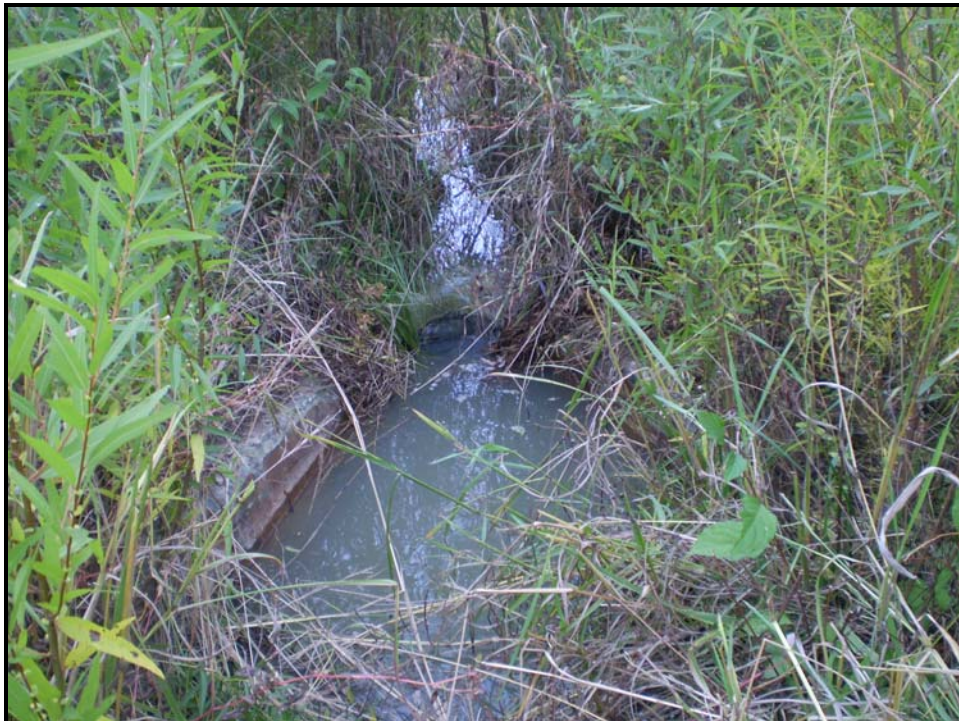
Stream Photo # 4 Rock Cross Vane Looking Upstream at Sta. 131+47
