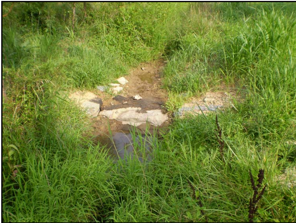
Stream Photo # 12 Boulder Sill Looking Upstream at Sta. 205+91
