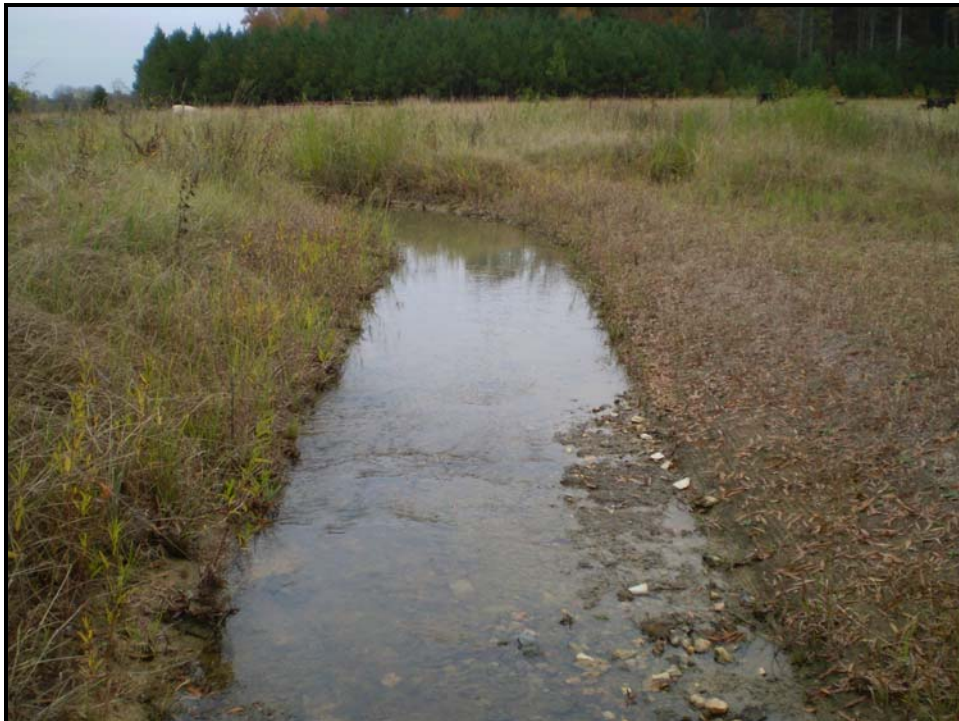
Stream Photo # 6 Constructed Riffle Looking Upstream at Sta. 137+80
