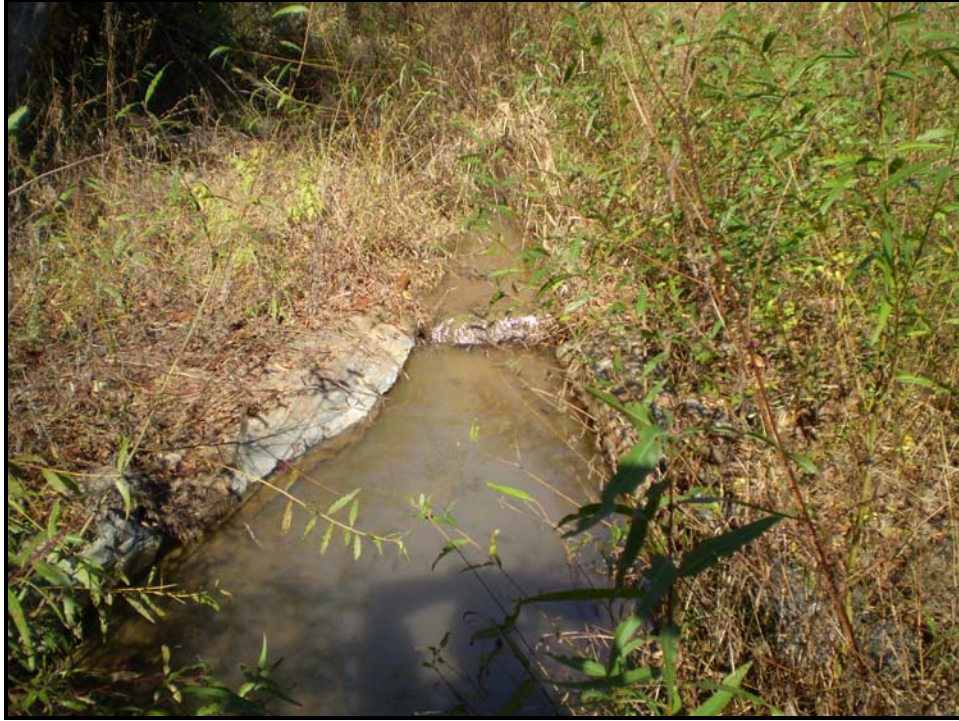
Stream Photo # 17 Rock Cross Vane Looking Upstream at Sta. 413+50
