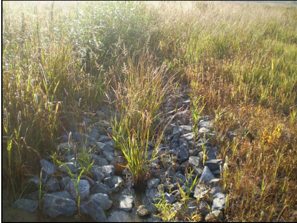
Stream Photo # 13 Constructed Riffle Looking Upstream at Sta.302+10
