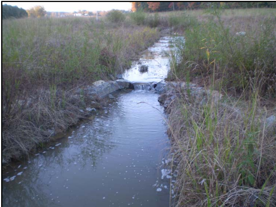
Stream Photo # 8 Rock Cross Vane Looking Upstream at Sta. 156+77
