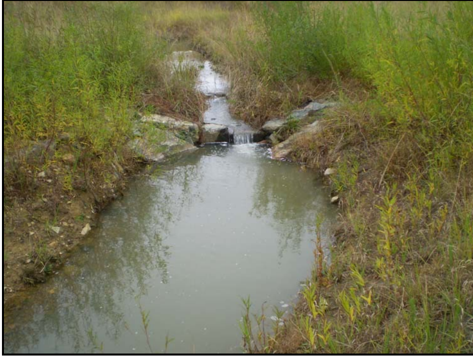
Stream Photo # 5 Rock Cross Vane Looking Upstream at Sta. 134+71
